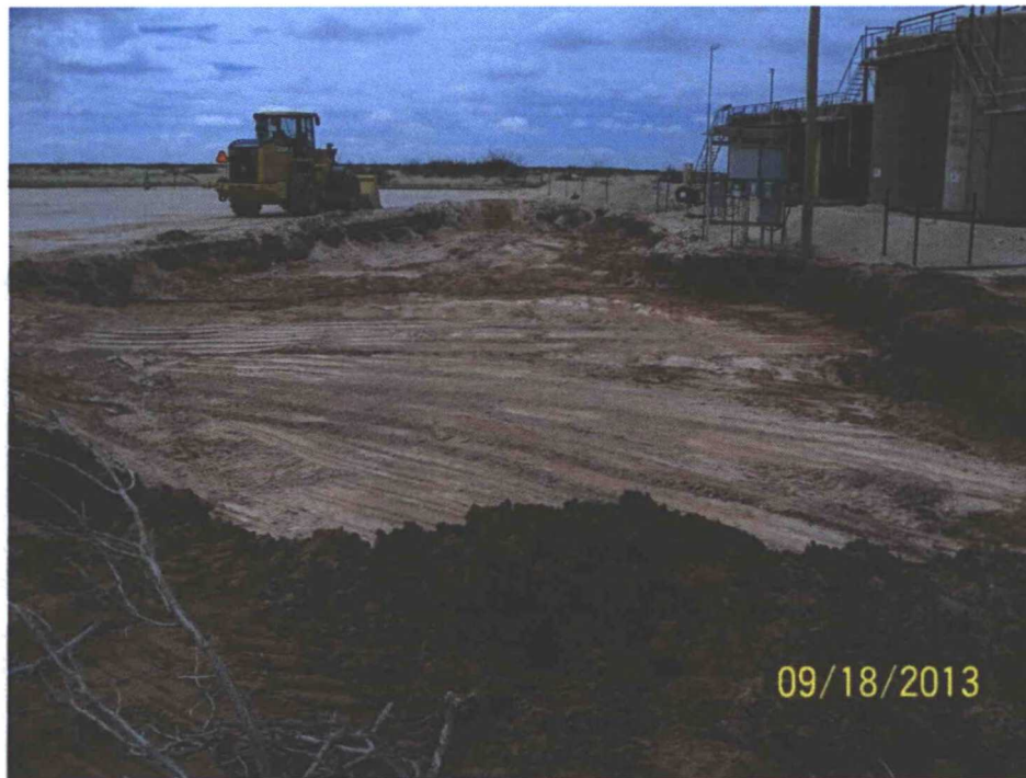
Photo 19: View of Excavated Release Area
