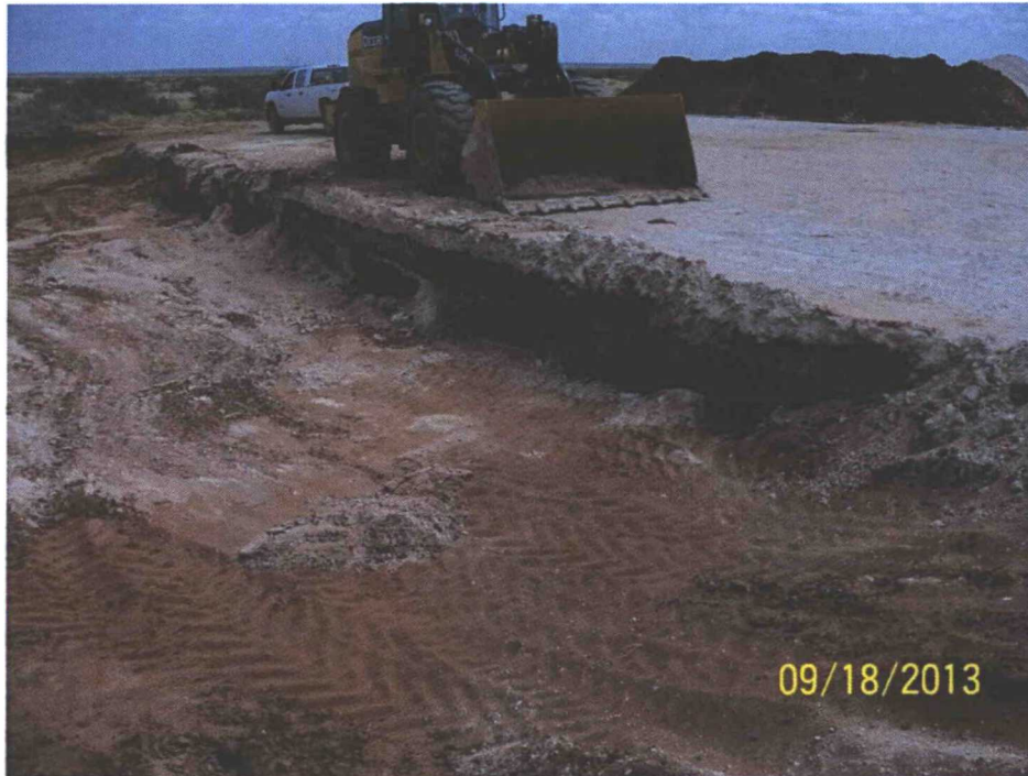
Photo 11: View of Excavation's South Wall near Southwest Corner
