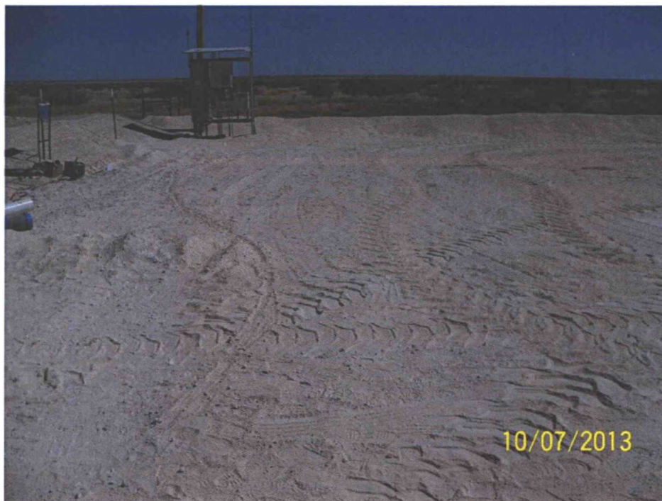
Photo 26: Another View of Backfilled and Compacted former Excavated Area on Facility's Pad
