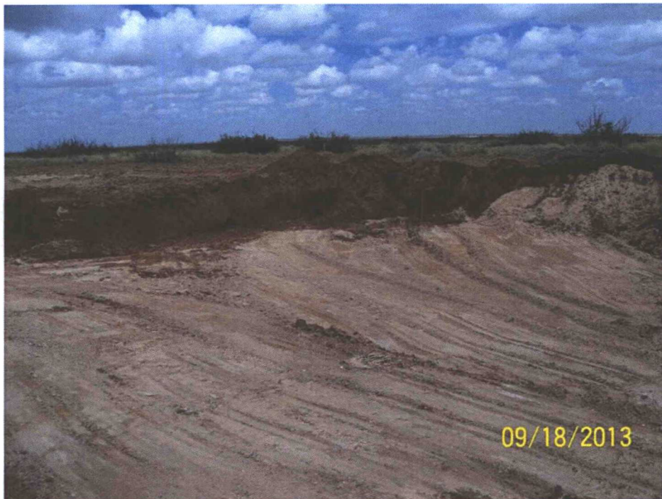
Photo 17: View of Excavation's Northeast Corner
