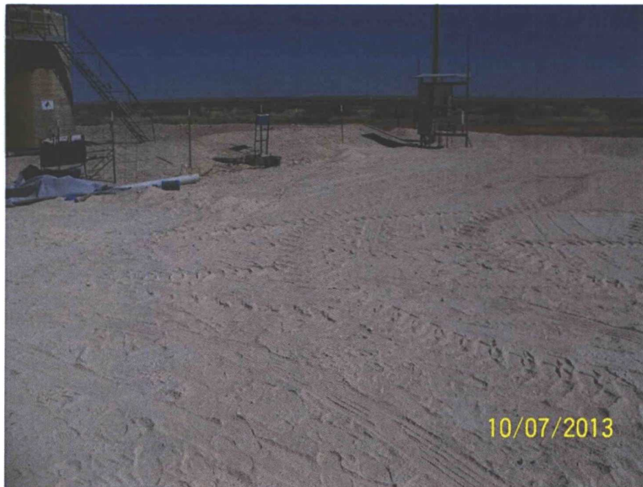
Photo 25: View of Backfilled and Compacted former Excavated Area on Facility Pad
