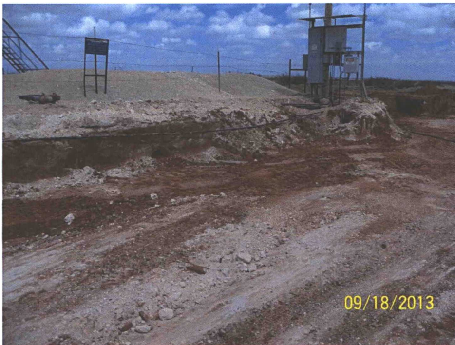
Photo 12: View of Excavation's North Wall of Excavation along Facility's Firewall
