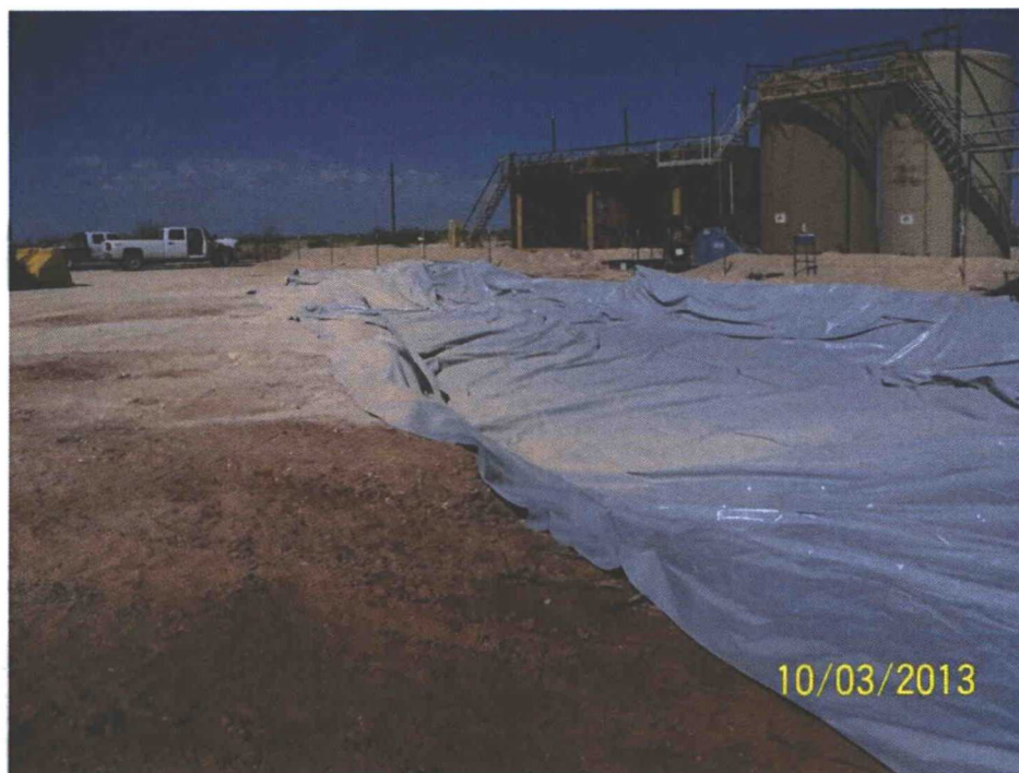
Photo 21: View of Liner installed in West Side of Excavation
