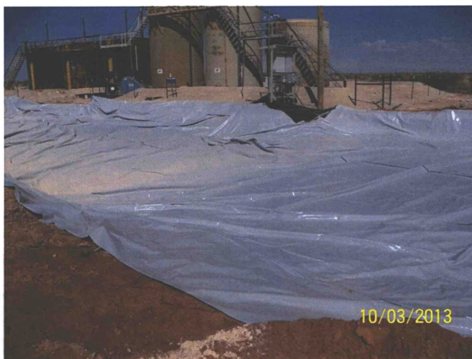
Photo 22: View of Liner in Center of Excavation
