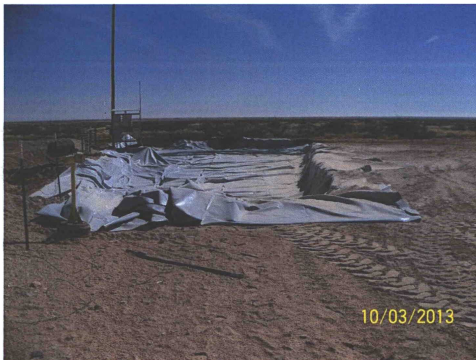
Photo 20: View of 20 mil Liner installed in Excavation
