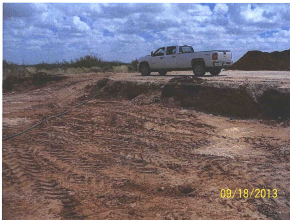
Photo 14: View of Excavation's South Wall near Southeast Corner
