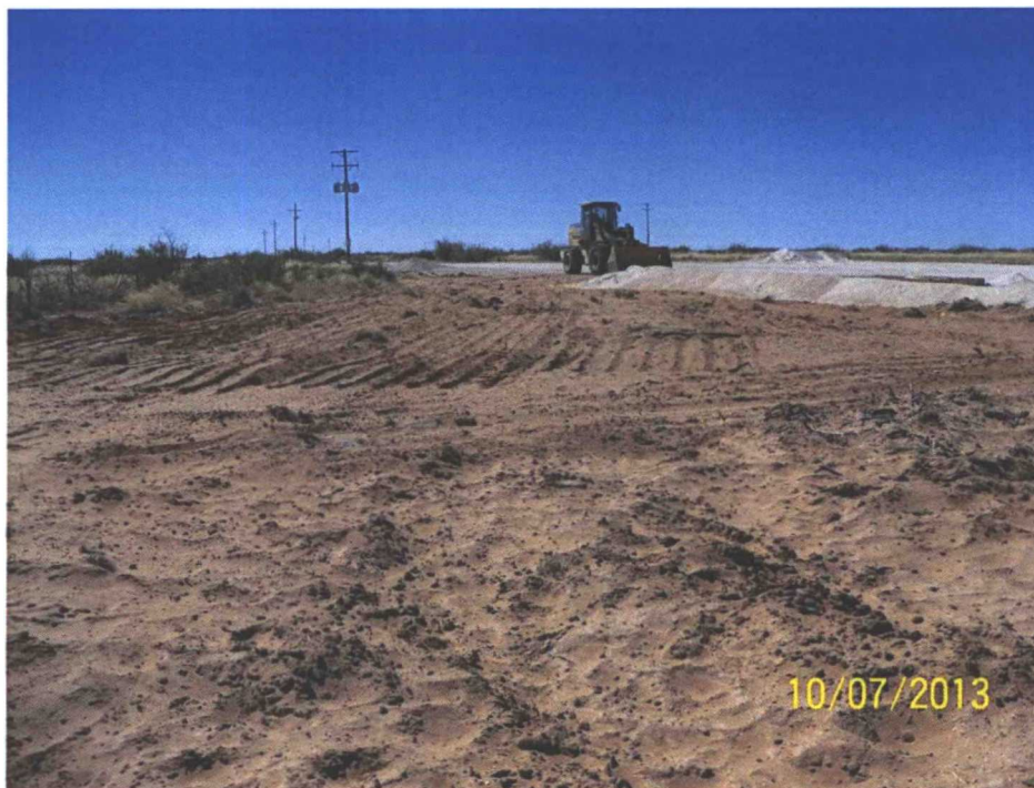
Photo 29: Another view of Contoured and Seeded Backfilled and Compacted former Excavated Area in Pastureland east of Facility's Pad
