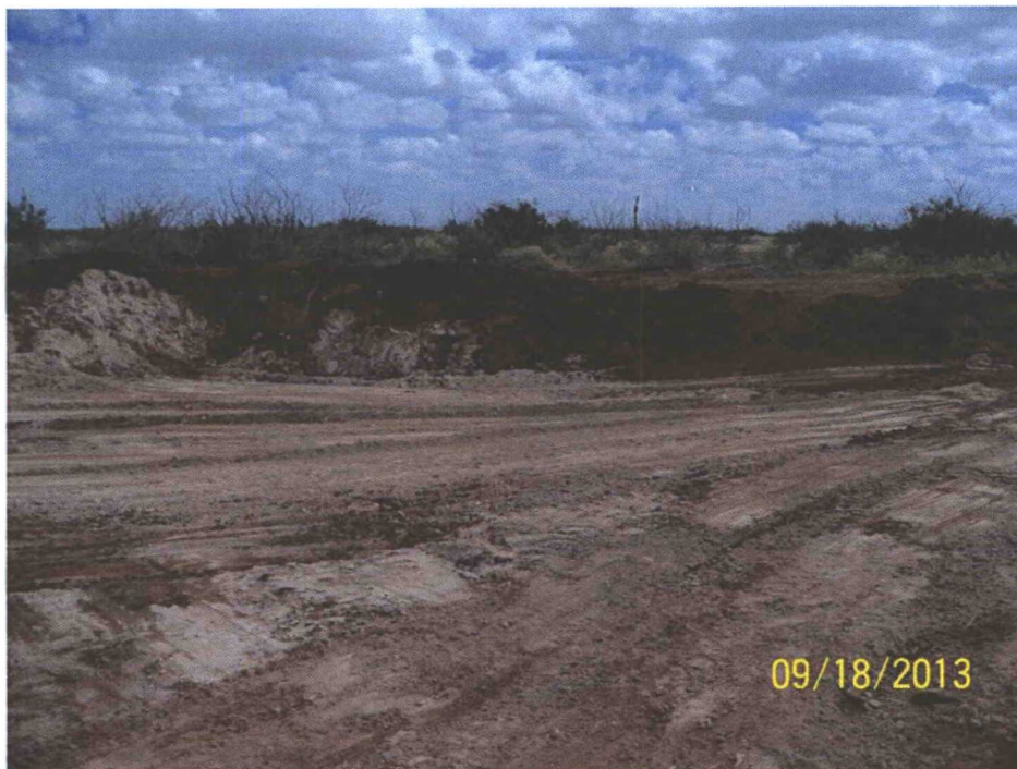
Photo 18: View of Excavation's Southeast Corner
