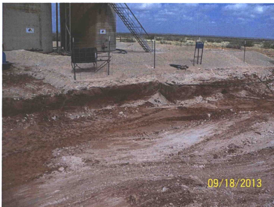
Photo 10: View of Excavation's North Wall along Facility's Firewall
