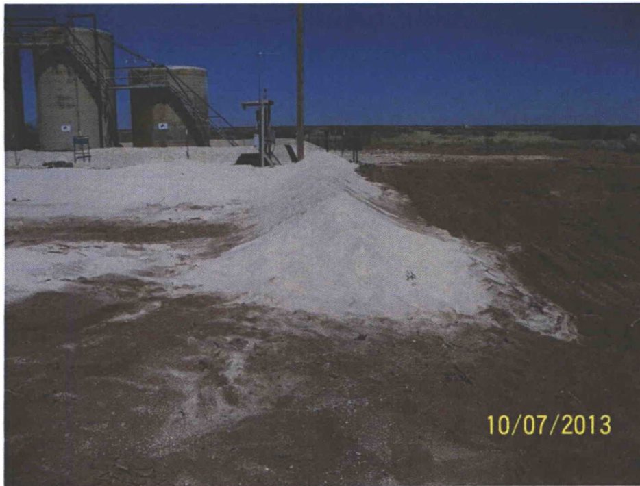
Photo 27: View of Diversion Berm constructed along eastern Edge of Facility's Pad
