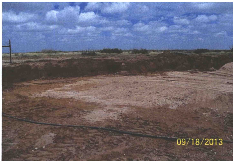
Photo 16: View of Excavation's North Wall near Northeast Corner
