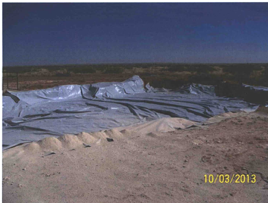
Photo 23: View of Liner installed in East Side of Excavation
