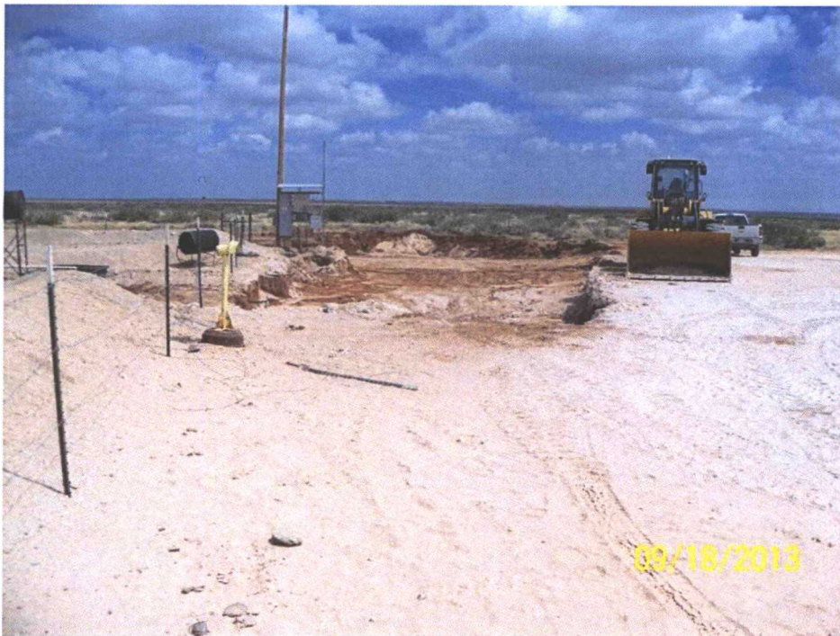
Photo 8: View of Excavated Release Area
