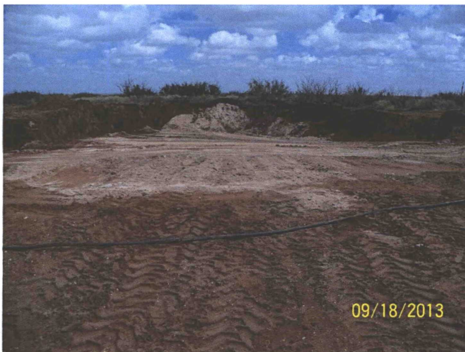
Photo 17: View of Excavation's East Wall
