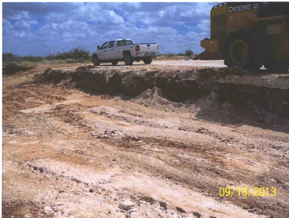
Photo 13: View of Excavation's South Wall Mid-Point
