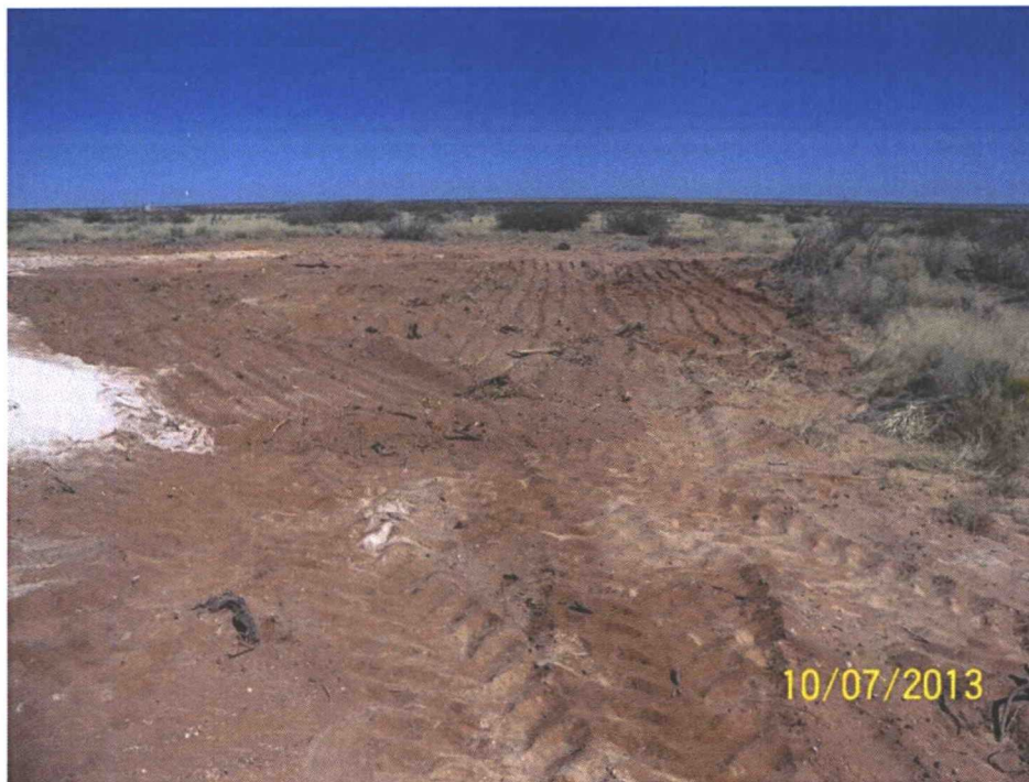
Photo 28: View of Contoured and Seeded Area on Backfilled and Compacted Former Excavated Area in Pastureland east of Facility's Pad
