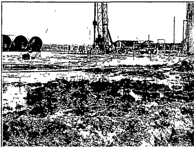
Figure 1. Soil berm used to limit surface migration of release soil and water.
