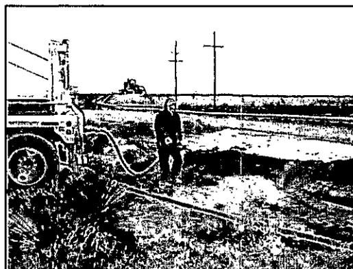
Figure 4. Example of suction hose being used to remove ponded water and oil.
