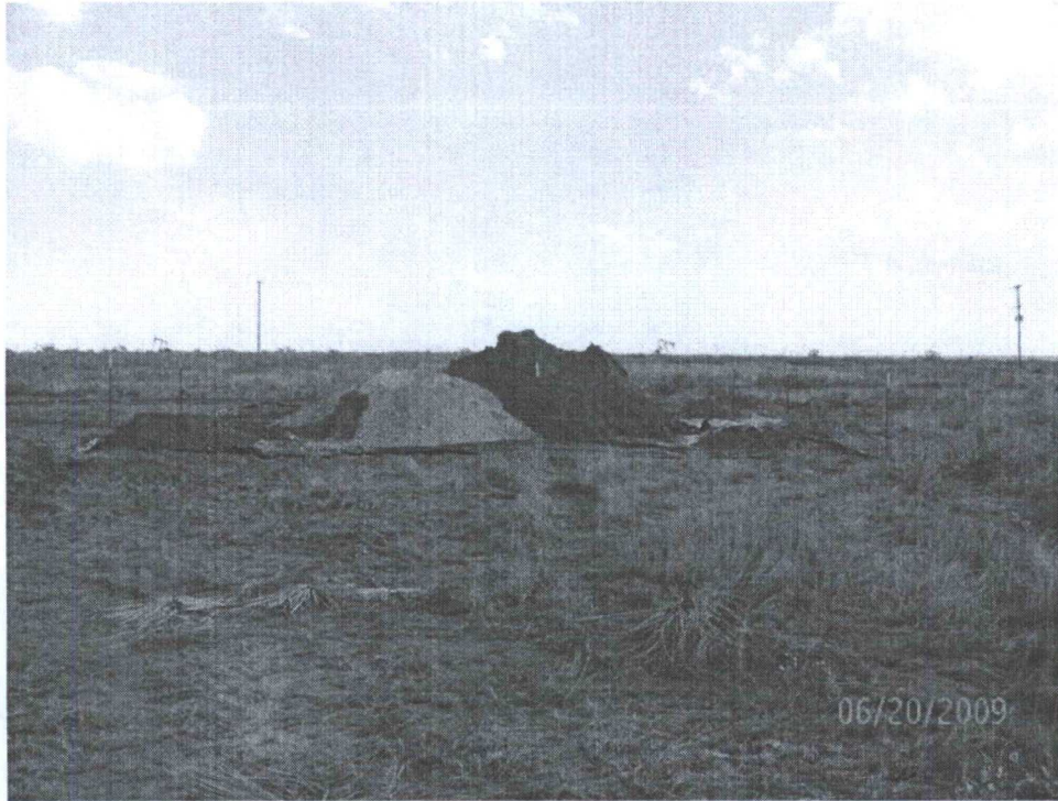
Photograph No. 3 – Impacted material stockpiled on plastic liners
