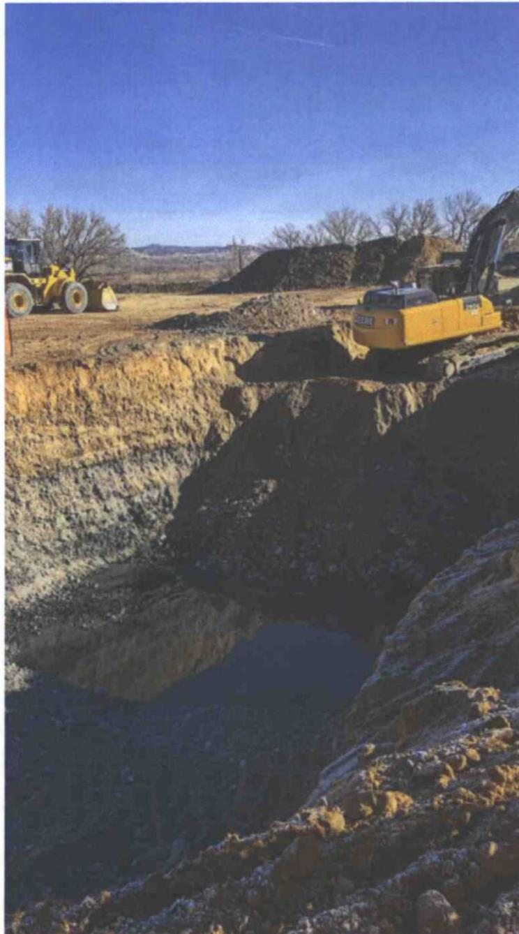
Photo 3 – Excavation with groundwater accumulation in eastern portion.
