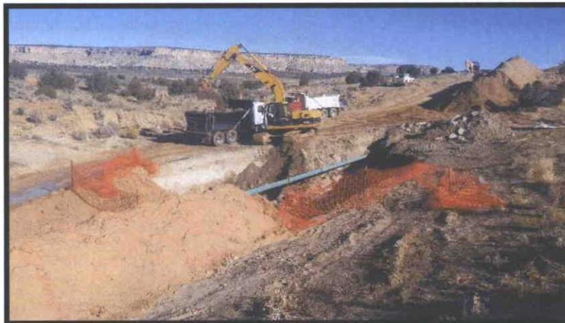
**Photo 8:** The October, 2015 2C-55 excavation nearing the final extents, just prior to sampling. Note dirty (gray) stockpile and clean imported (red and tan) backfill stockpiles in background.
