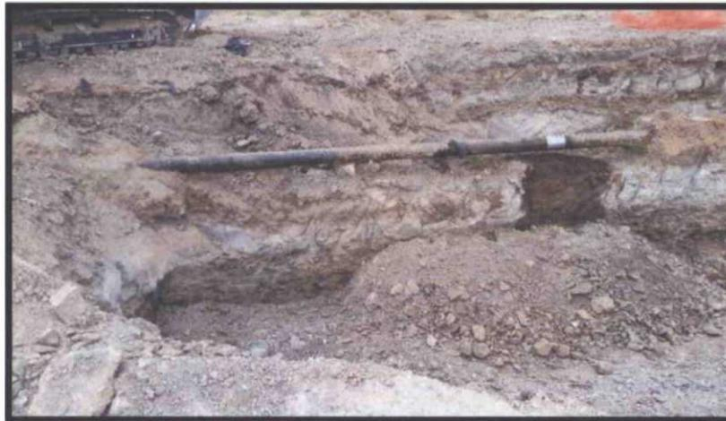
**Photo 4:** A temporary clamp was installed to prevent further contamination and to allow the requisite pre-repair activities to take place.
