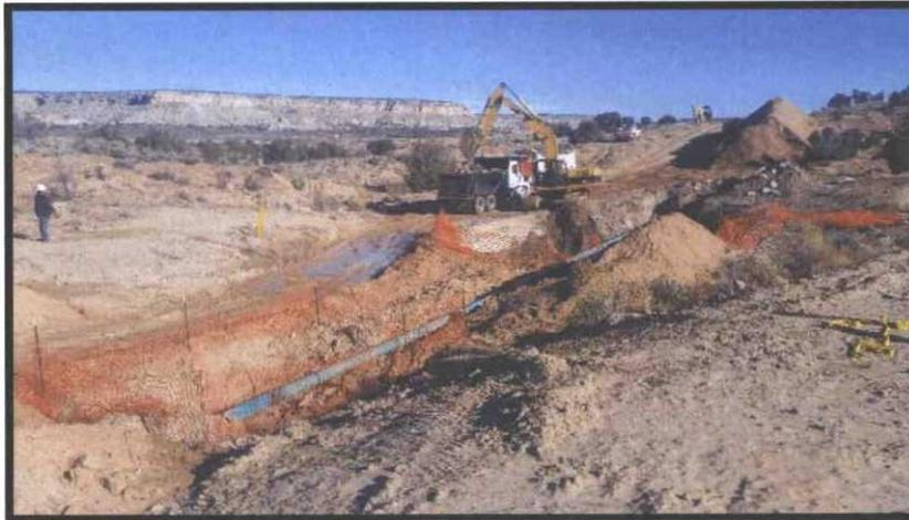
**Photo 7:** Excavation of the remaining contaminated soils after repair activities concluded.
