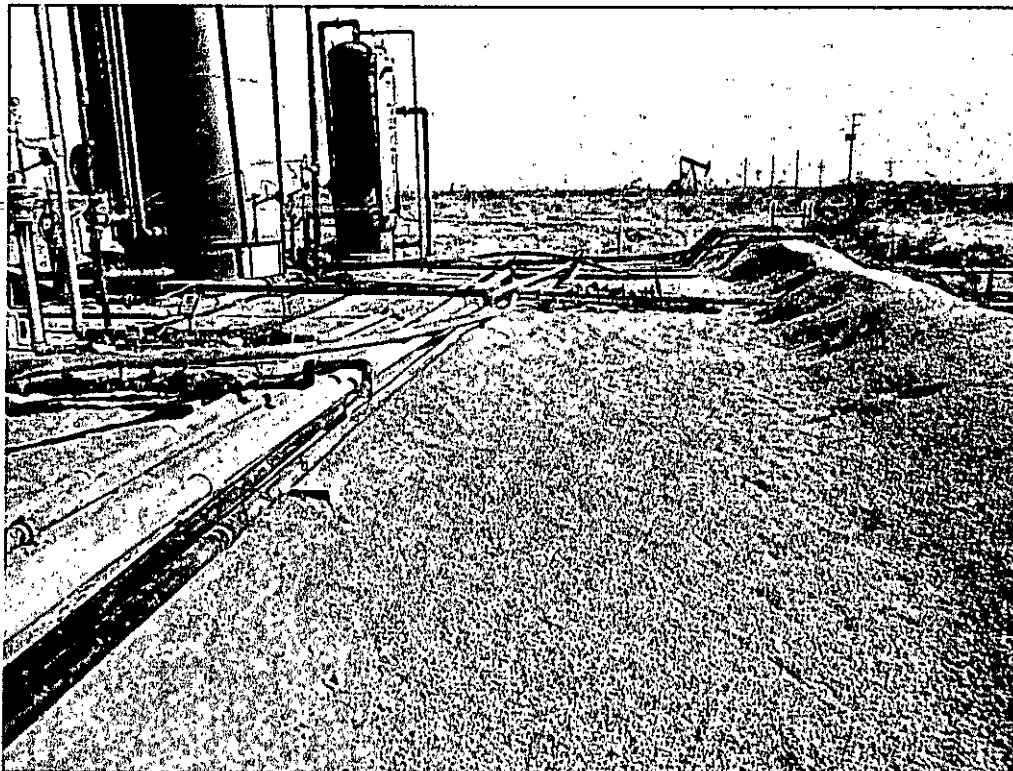
Backfill topped with gravel
