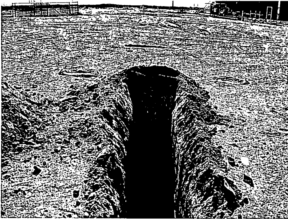
Typical Backhoe Trench
