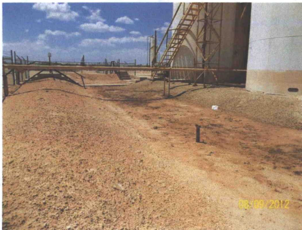
Photo 2. View looking west at spill area with AH-5 and AH-6.
