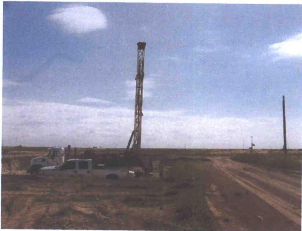
View East– Area of SB-1 (AH-4)
