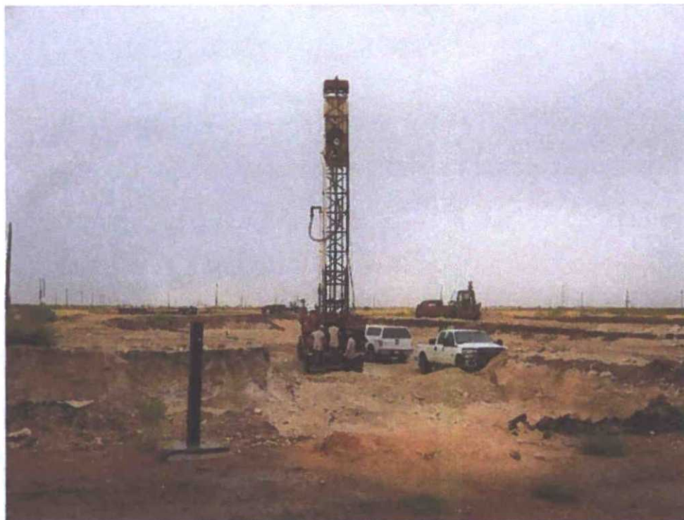
View West – Area of SB-2 (AH-10)
