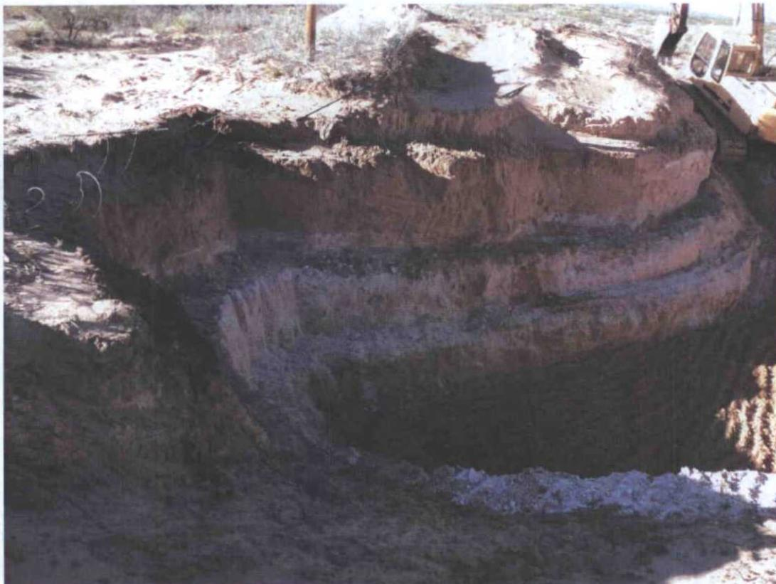
**Photograph No. 1 - Looking westerly at excavation, benching and sidewall overburden**
