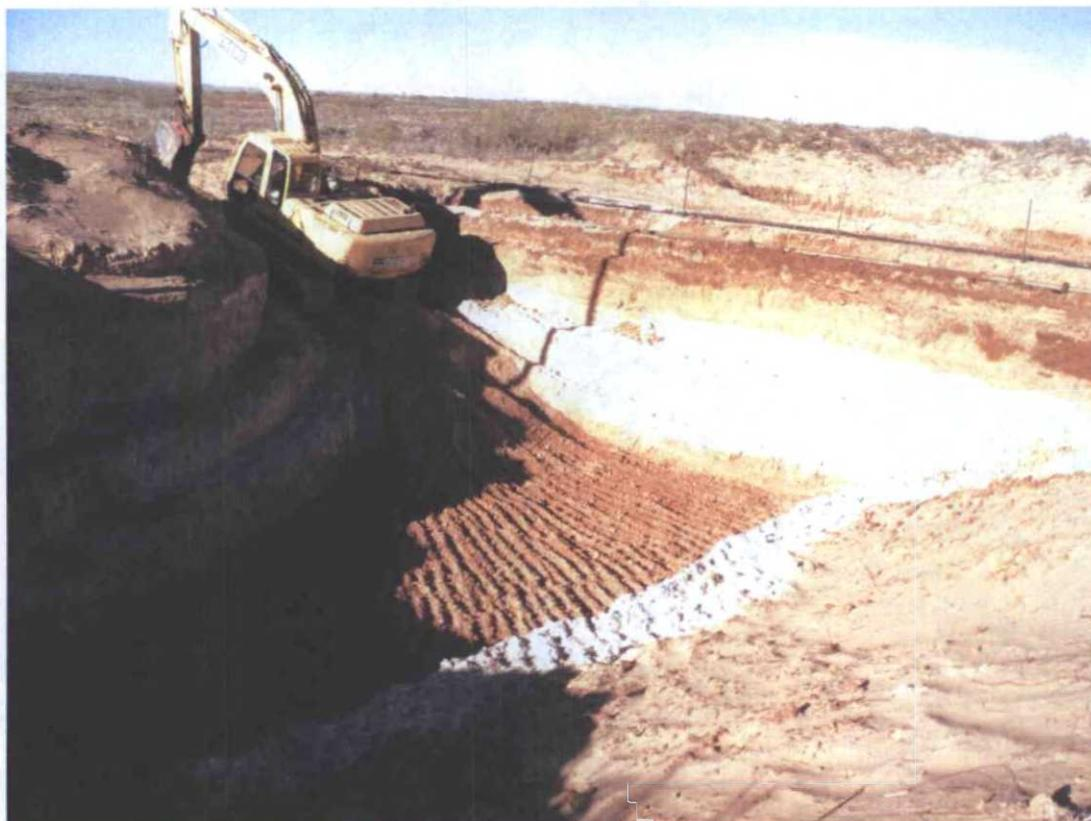
**Photograph No. 2 - Looking westerly at ingress/egress ramp, excavation, flow lines, benching and sidewall overburden**
