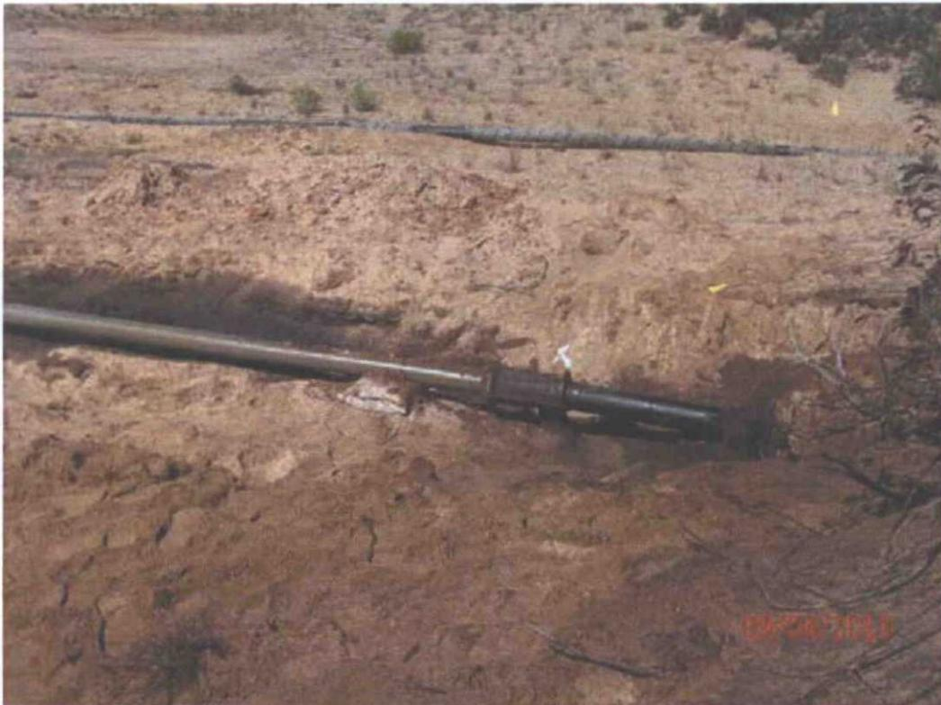
Photograph No. 4 – Looking at Point of Release and repair clamp
