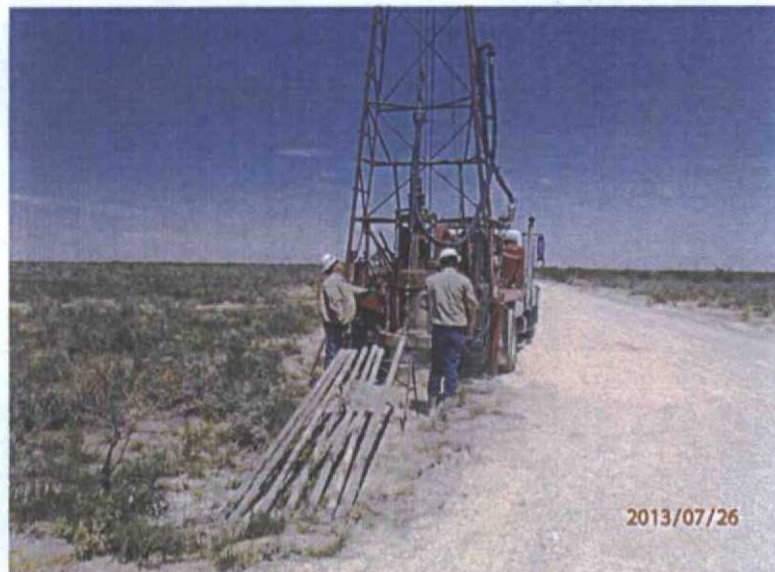
Installing temporary MW, facing east
