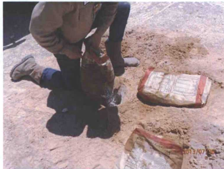
Plugging soil bore #1 in total with bentonite
