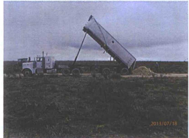
Import caliche to build surface for soil bore installations facing, west
