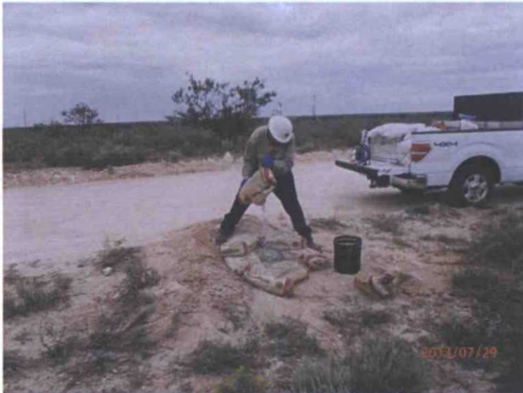
Plugging temporary MW in total with bentonite, facing southwest 7/29/13
