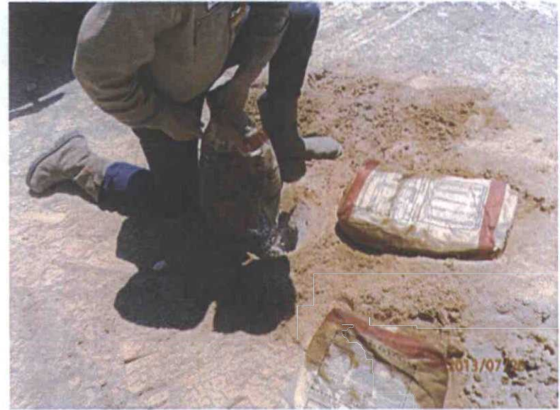
Plugging soil bore #1 in total with bentonite
