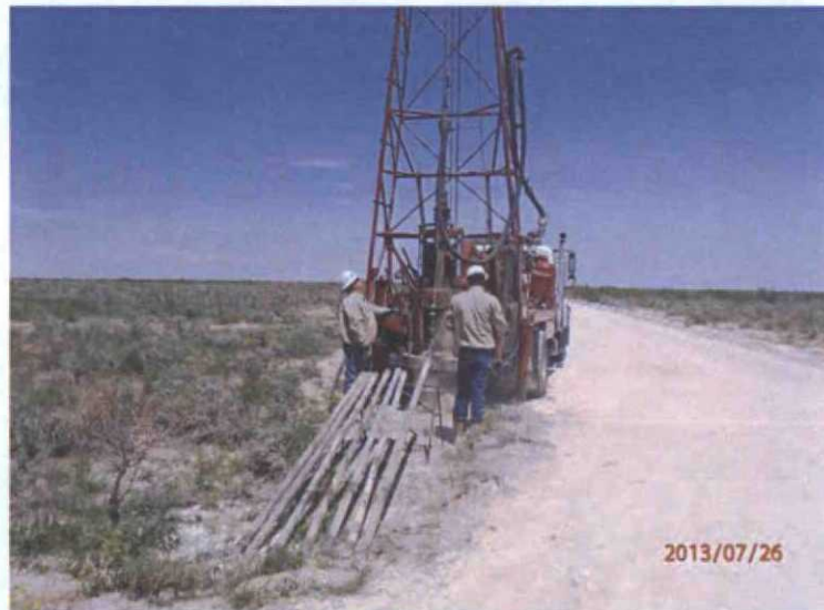
Installing temporary MW, facing east
