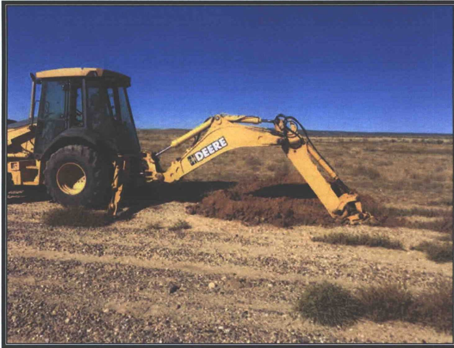
Photo 17: Trench for Sump Investigation
