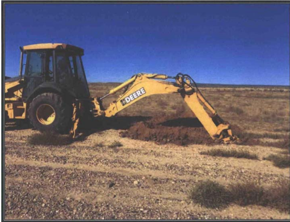
Photo 17: Trench for Sump Investigation
