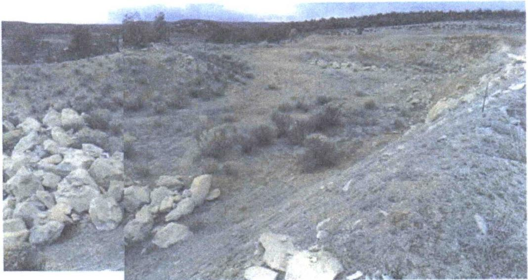
*View north of proposed site. To the left, out of the photograph, is a restored and vegetated portion of the former rock quarry site. Placing drill cuttings in the former quarry will help restore original topography.*
