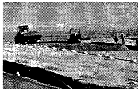
Capillary Barrier Installation
