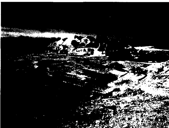
Figure 6: Place coarse-grained material over 5% slope
