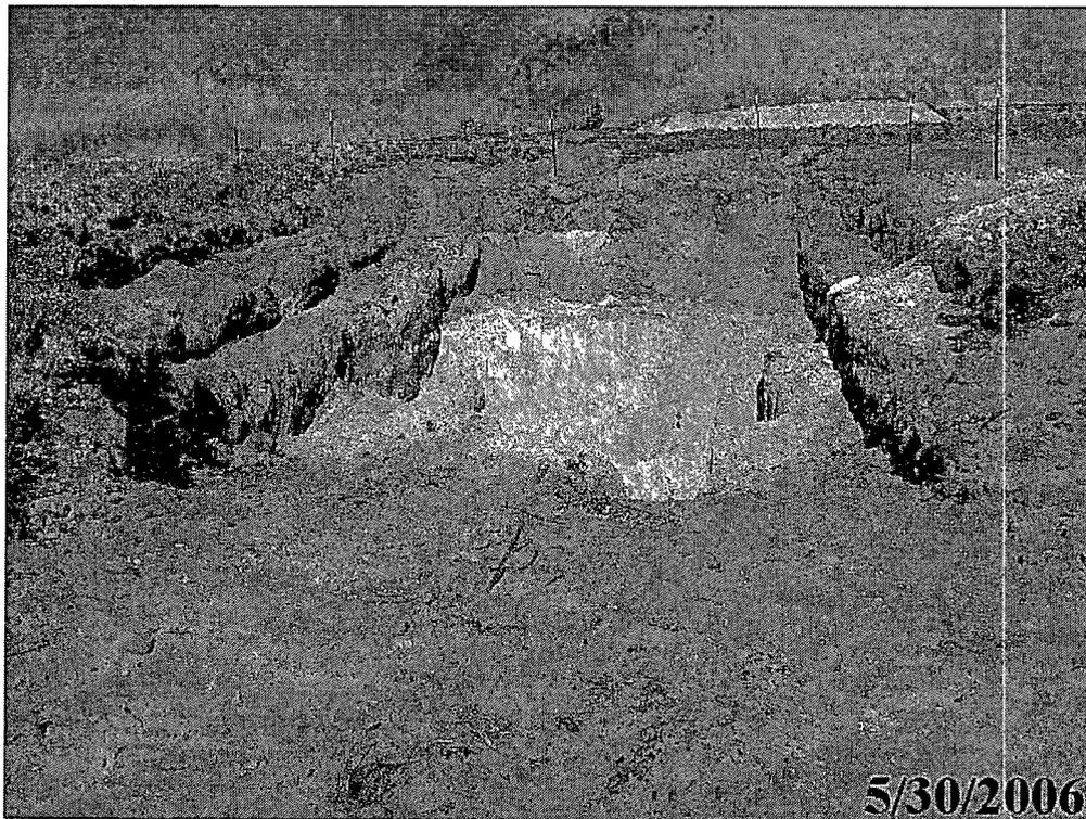
**Photograph #2** – Looking westerly across Site #4 excavation. Orange pin flags on excavation sidewalls and floor indicate soil sample locations.
