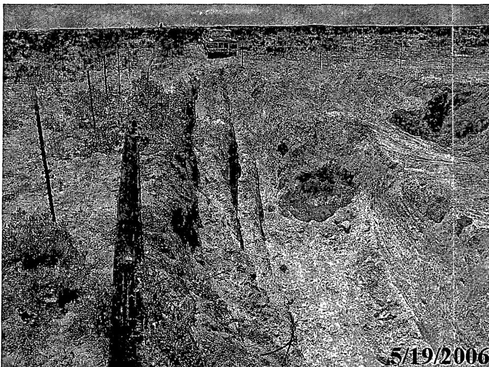
**Photograph #2** – Looking westerly at Site #2 excavation. Orange pin flags on excavation sidewalls and floor indicate soil sample locations.
