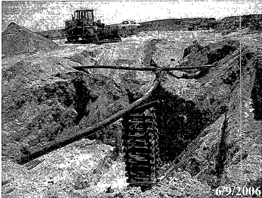
**Photograph #3** – Looking easterly at Site #1 excavation. Orange pin flags on excavation sidewalls and floor indicate soil sample locations.
