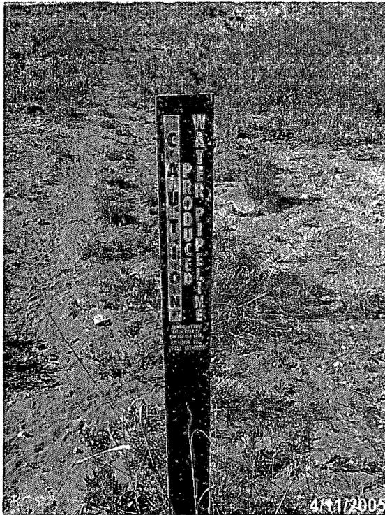
Photograph #1 – Produced water pipeline ROW marker
