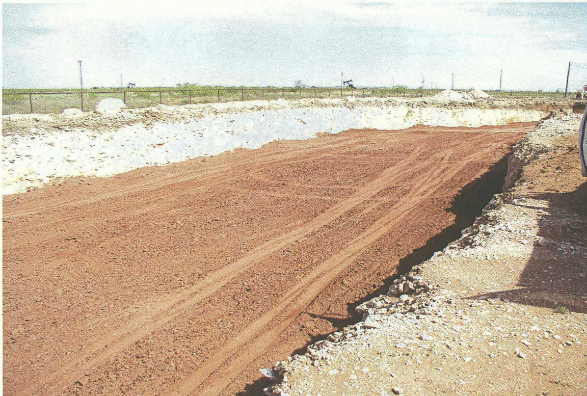
No. 74 – View of clay placed in the northeast excavation area.
