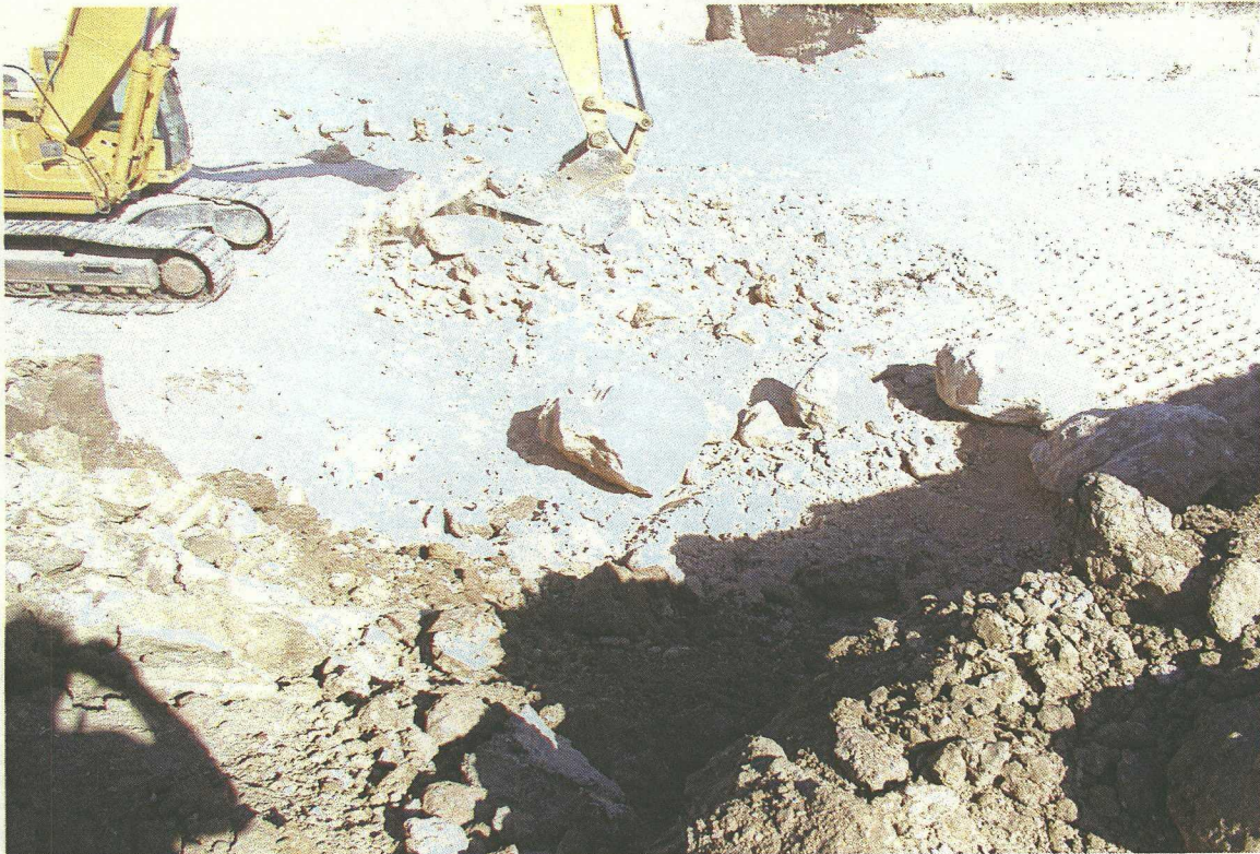
No. 63 – View of cobble cluster being broken in order for the cobbles to be removed from the excavation.
