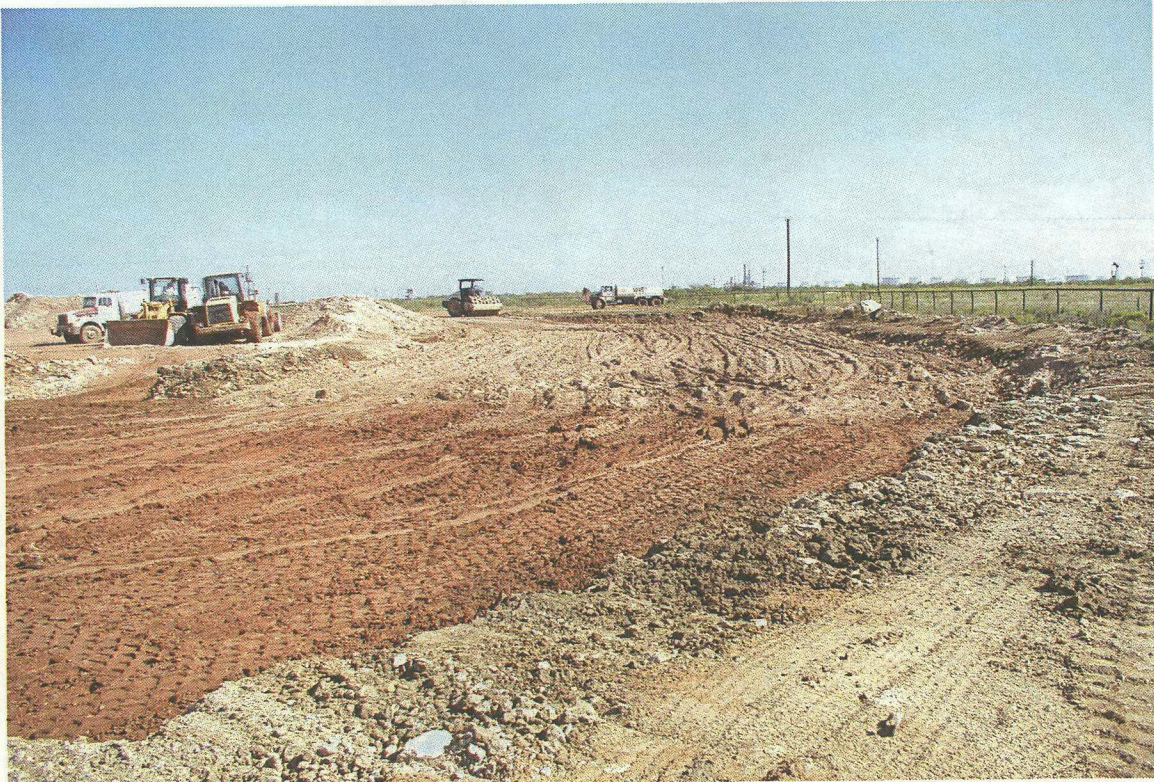
No. 103 – View of the initial placement of the caliche.
