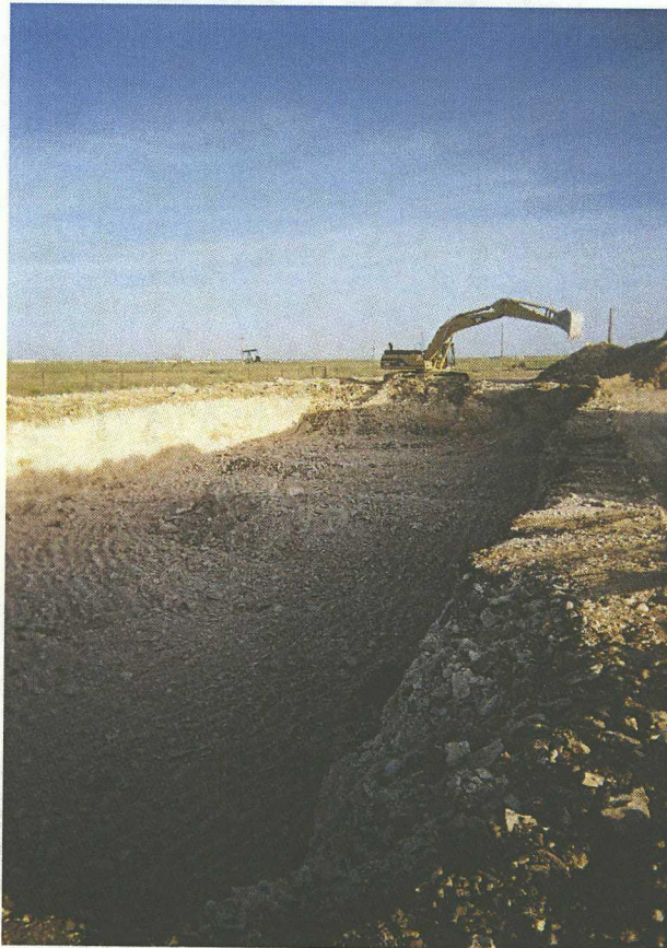
No. 22 – Northeastern part of the excavation with view of hard rock area that was not removed.
