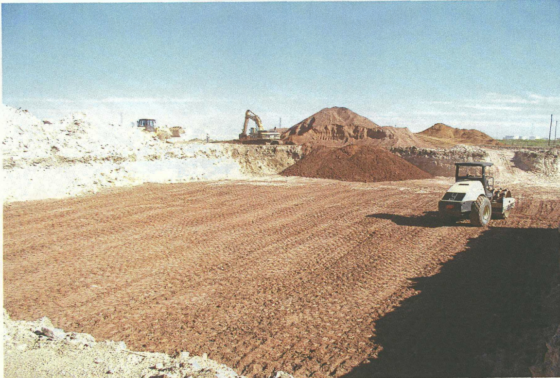
No. 69 – View of the beginning of the placement of the clay in the excavation.
