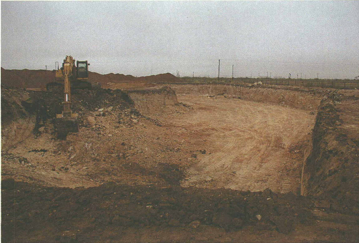
No. 35 – View of heavy petroleum staining at the location of former aboveground storage tanks (ASTs).
