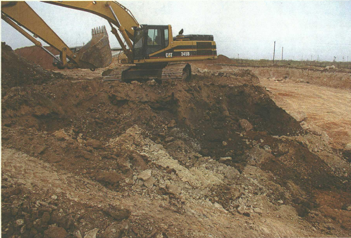
No. 33 – View of the excavation continuing and exposing relic piping. The piping was removed and disposed of as construction debris.
