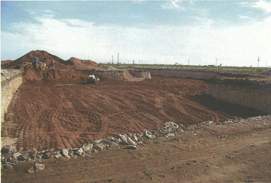
No. 73 – View of the placement of the first foot of clay across the entire base of excavation.
