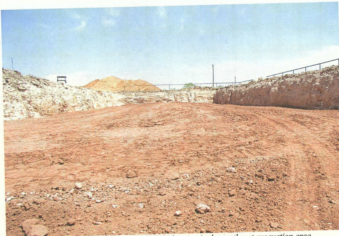
No. 81 – View of the beginning of the 4% grade forming in the northeast excavation area.
