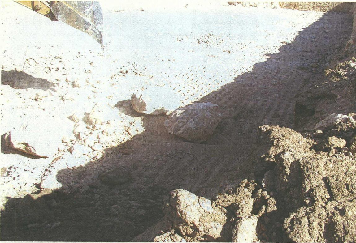
No. 65 – View of the sheep-foot roller marks left after preparing the bottom of the excavation for backfill.
