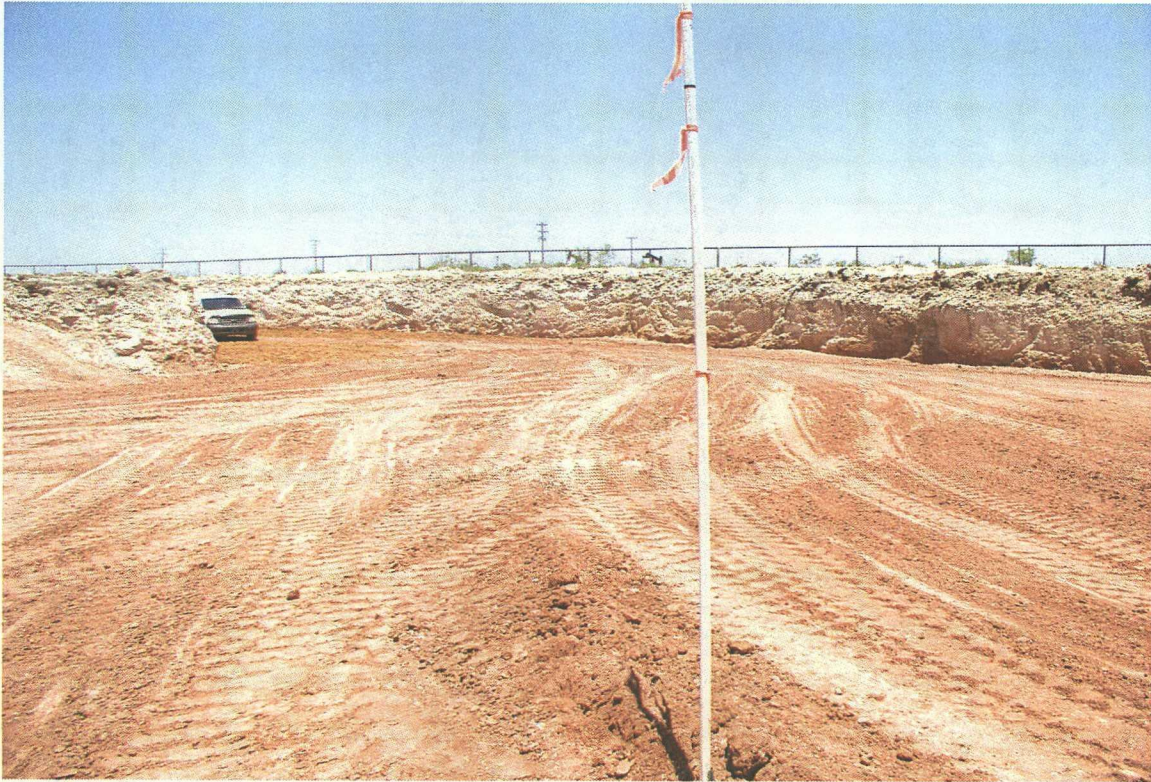
No. 93 – View of the grade marker where clay is almost four feet thick from the farthest point along the 4% grade.
