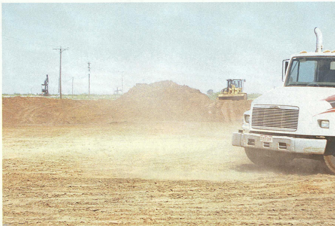
No. 100– View of the compacted sand material in the large excavation area after removal of the sheep-foot roller.
