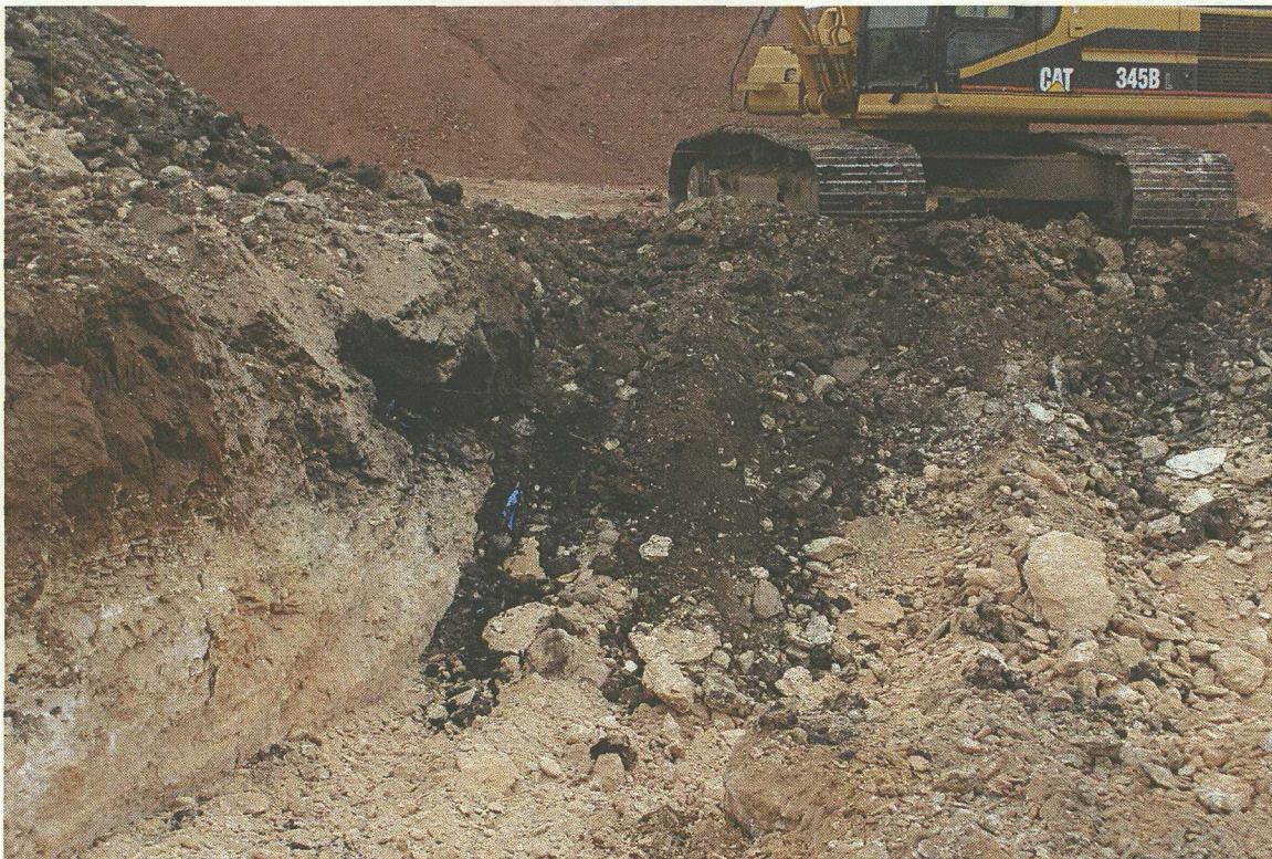
No. 36 – View of soil staining. The blue color is from buried PVC piping as it is exposed.
