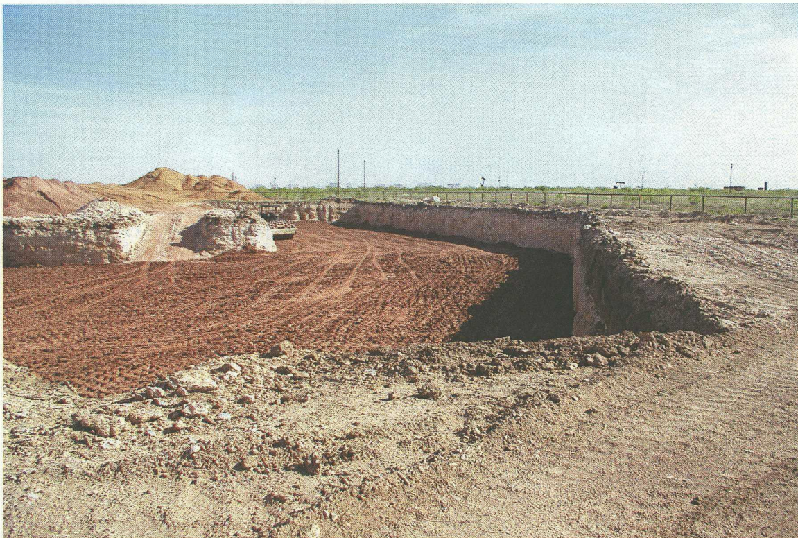
No. 78 – View of the base of the excavation with one-foot of clay placed.
