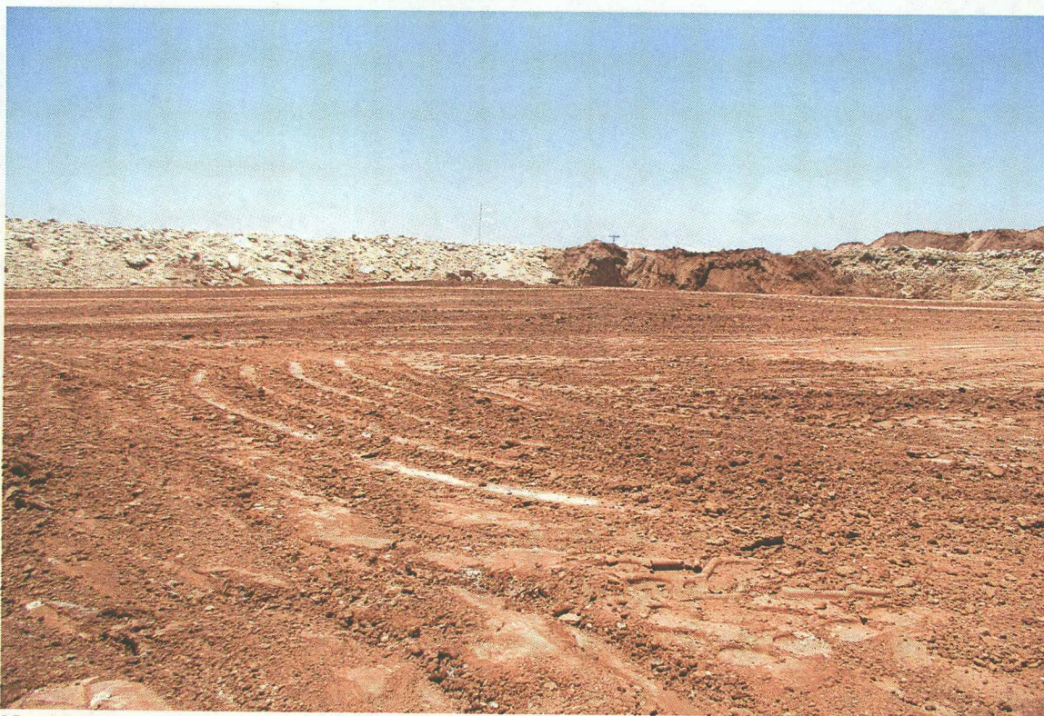
No .90 – View of the clay cap continuing to be installed in the large excavation area.
