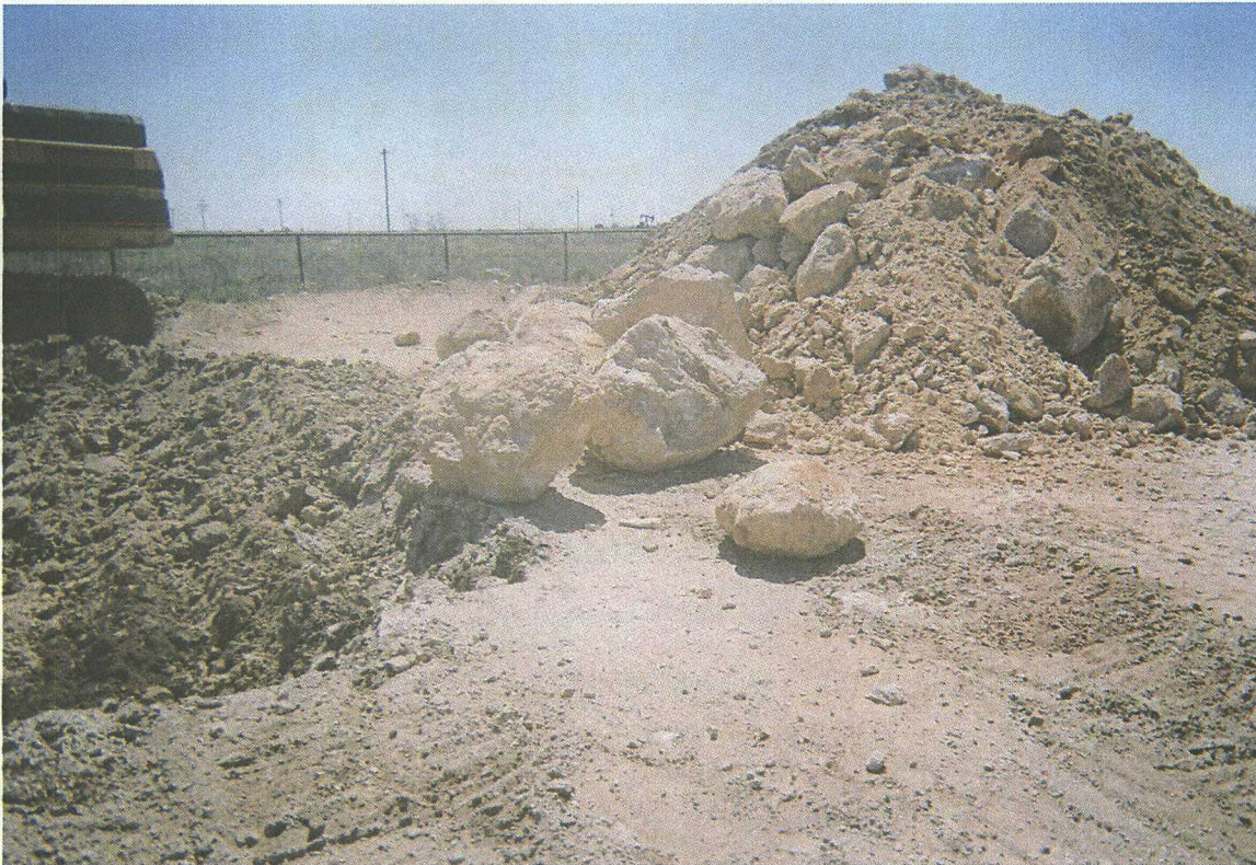
No. 13 – View of very large cobbles not able to be broken loose in the excavation.
