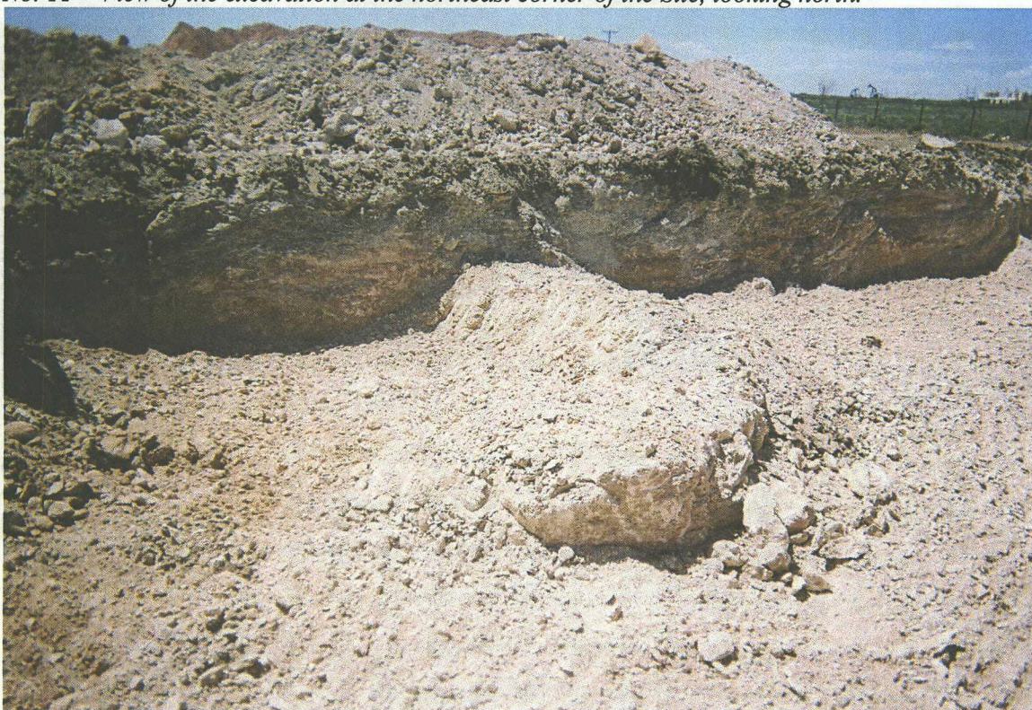
No. 12 – View of an encountered hard rock that could not be removed from the excavation.
