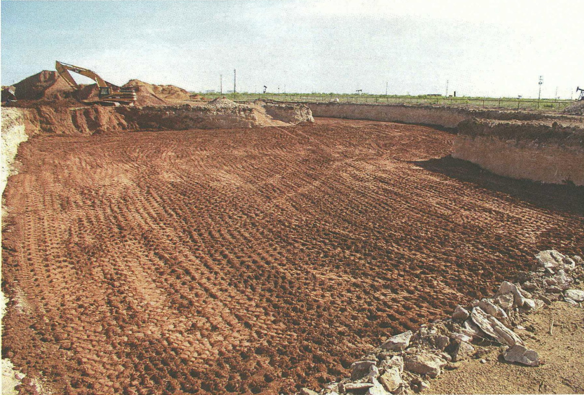
No. 77– View of the clay after compaction.
