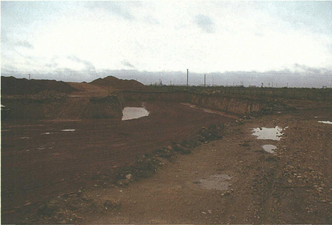
No. 85 – View of the water draining into the excavation from the ramp (left side of picture) and the water entering as rainfall (on the right side of the picture).
