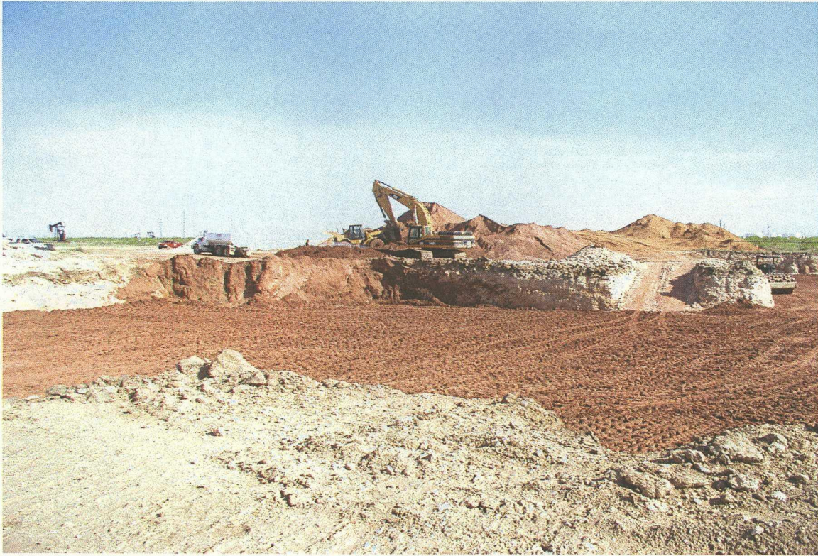
No. 79 – View of the clay processing (dumped in the corner of excavation for later spreading by the front-end loader).
