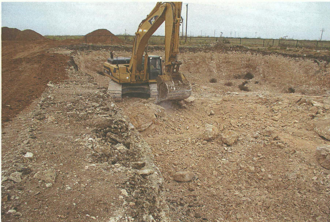
No. 30 – View of the excavator breaking up the cobble clusters.
