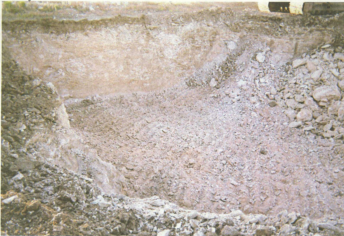
No. 4 – View of loose soil at the surface. Most of the digging is through hard caliche.
