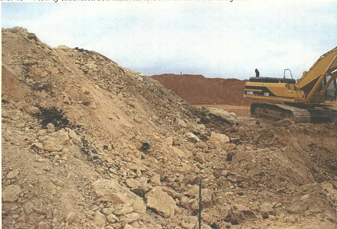
No. 44– View of excavated soil material to be removed to the landfarm (imported clay material is stockpiled in the background).
