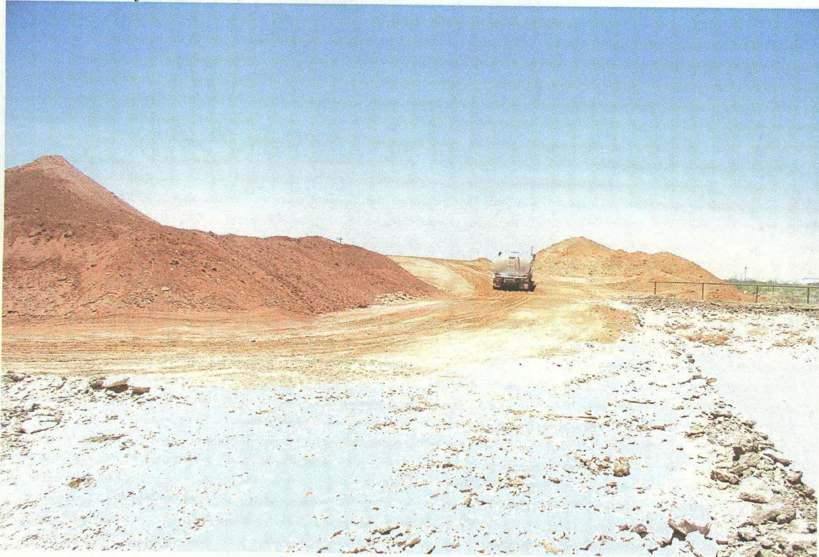
No. 62 – View of dust control methods.
