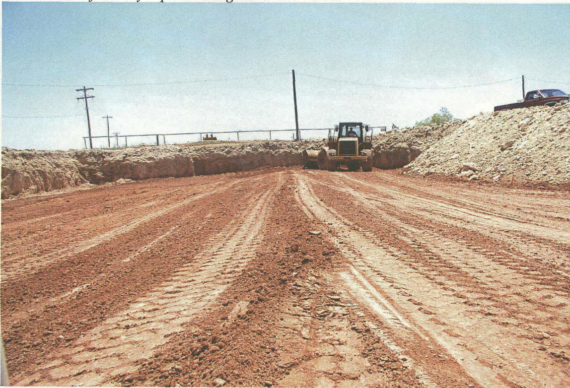
No. 92 – View of constructing the crown at the transition from the northeast excavation area to the large excavation area.
