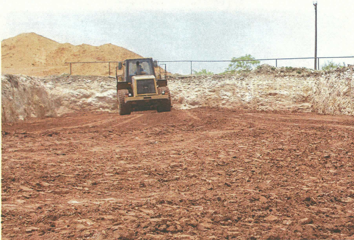
No. 83 – View of the clay cap in the northeast excavation area as it is completed.
