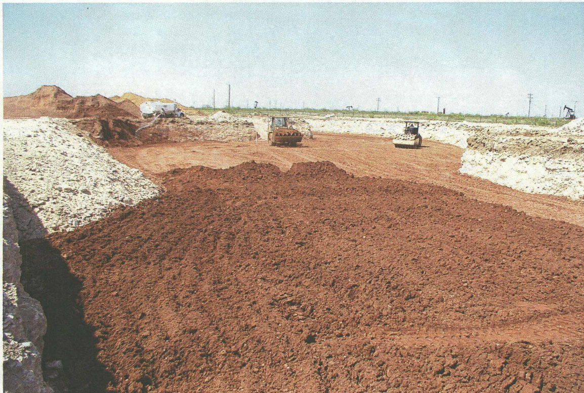
No. 84 – View of the 4% grade in the northeast excavation area as it is completed.
