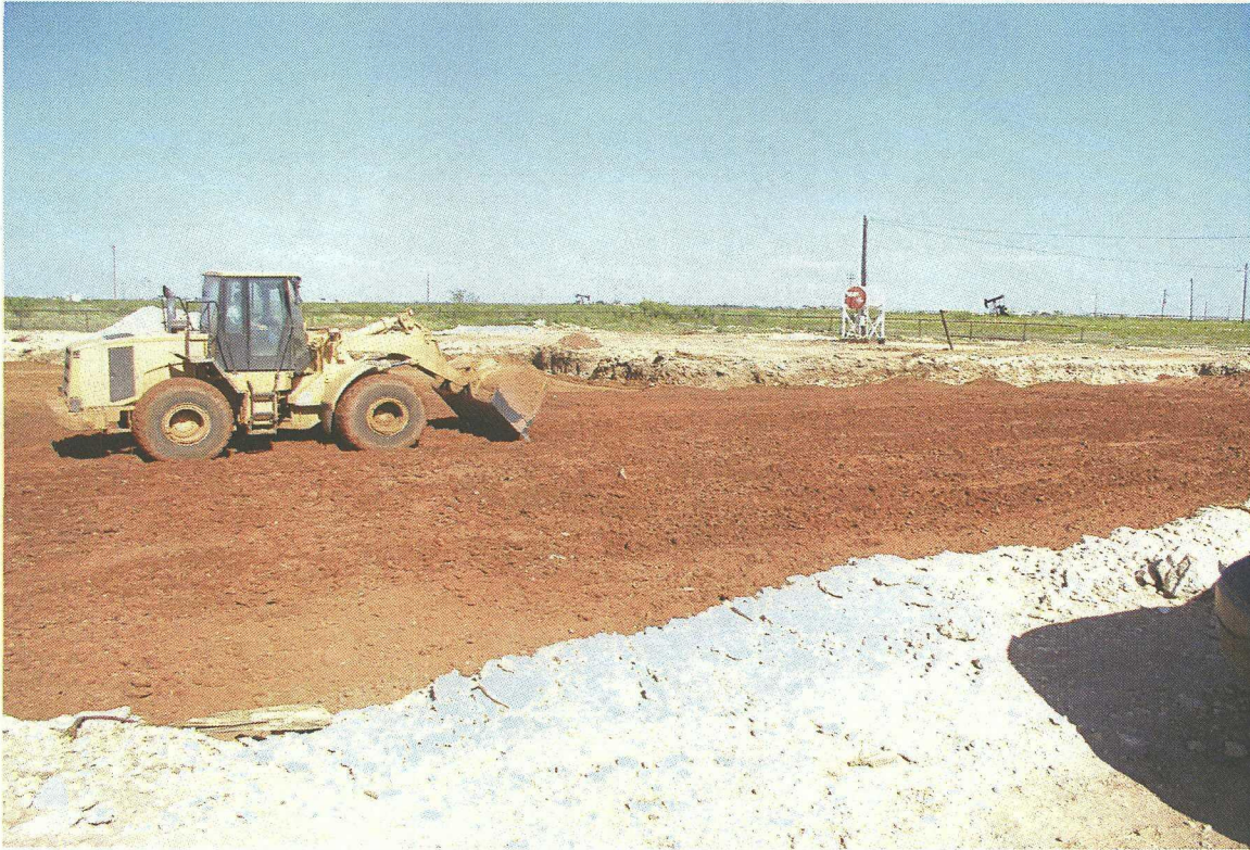
No. 101 – View of the placement of the sand lift within the large excavation area.
