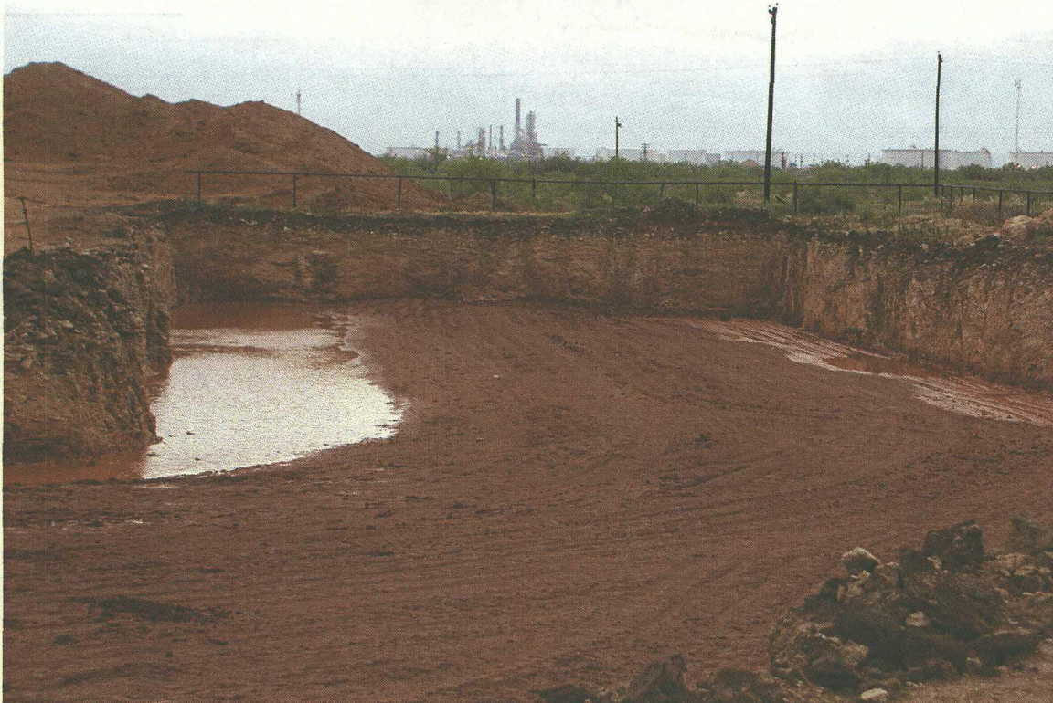
No. 86 – View of the water ponding within the northeast excavation area after clay cap placement.
