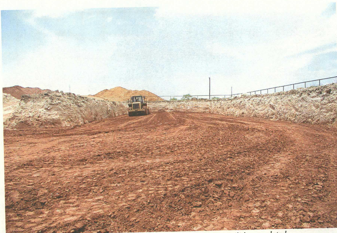
No. 82 – View of the 4% grade in the northeast excavation area as it is completed.
