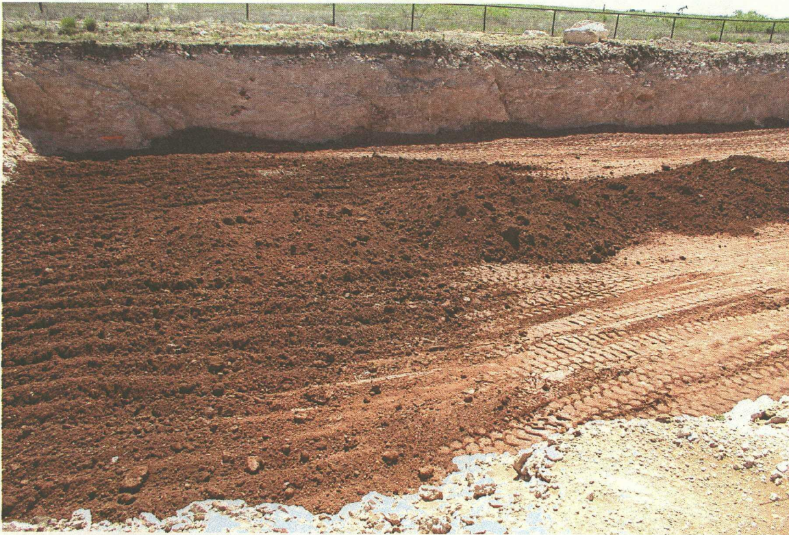
No. 80– View of the 4% slope of the clay cap in the northeast excavation area.
