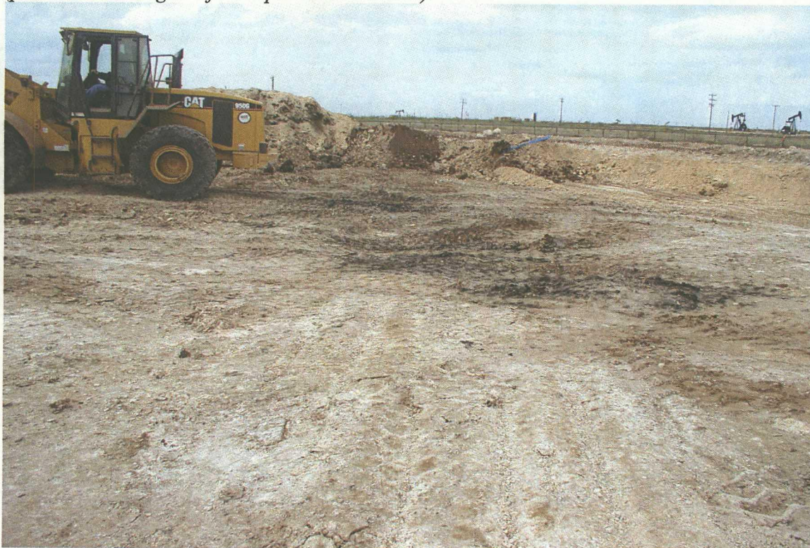
No. 46 – While loading trucks with soil material, staining would surface from vehicle traffic and soft spots in the surface soils would develop.
