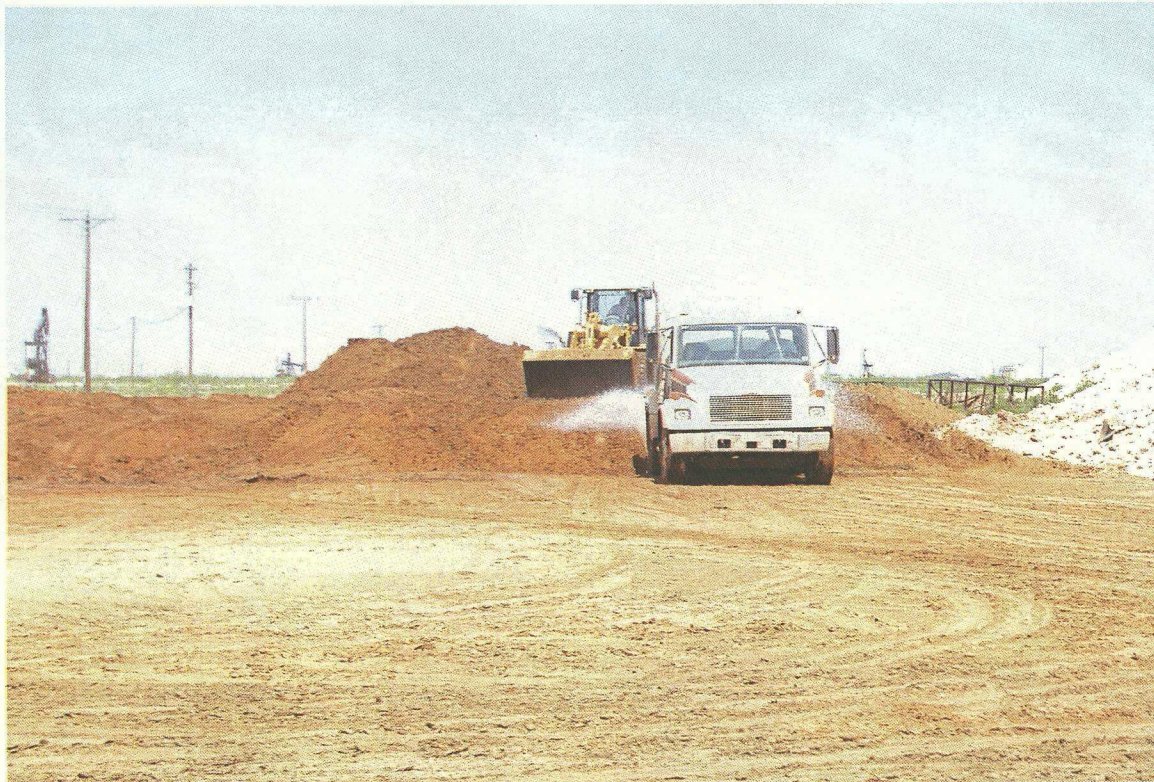
No. 99 – View of the watering and compaction of the sand material in the large excavation area.
