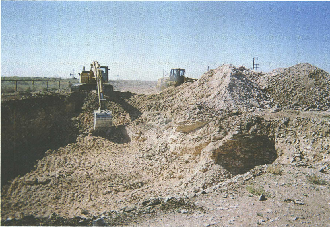
No. 3 – View of hard-digging, with the excavated material being stockpiled for loading trucks to the landfarm.
