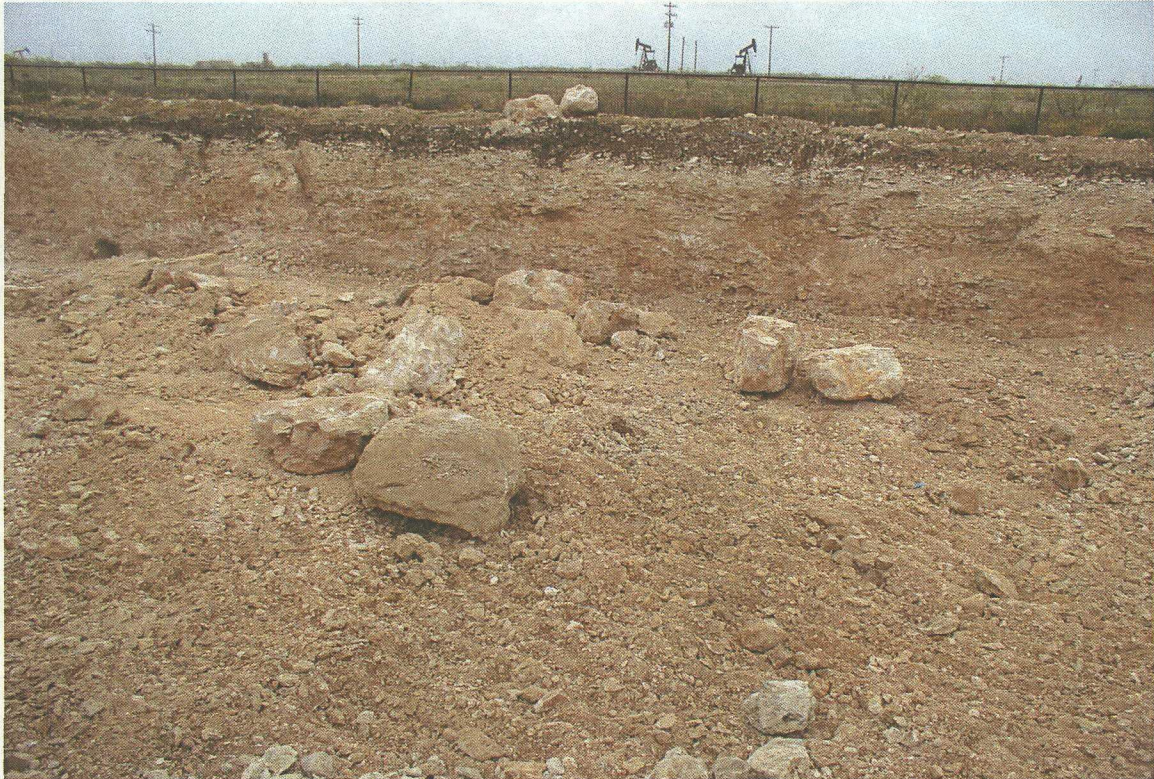
No. 29 – View of large cobbles encountered in various places within the excavation.
