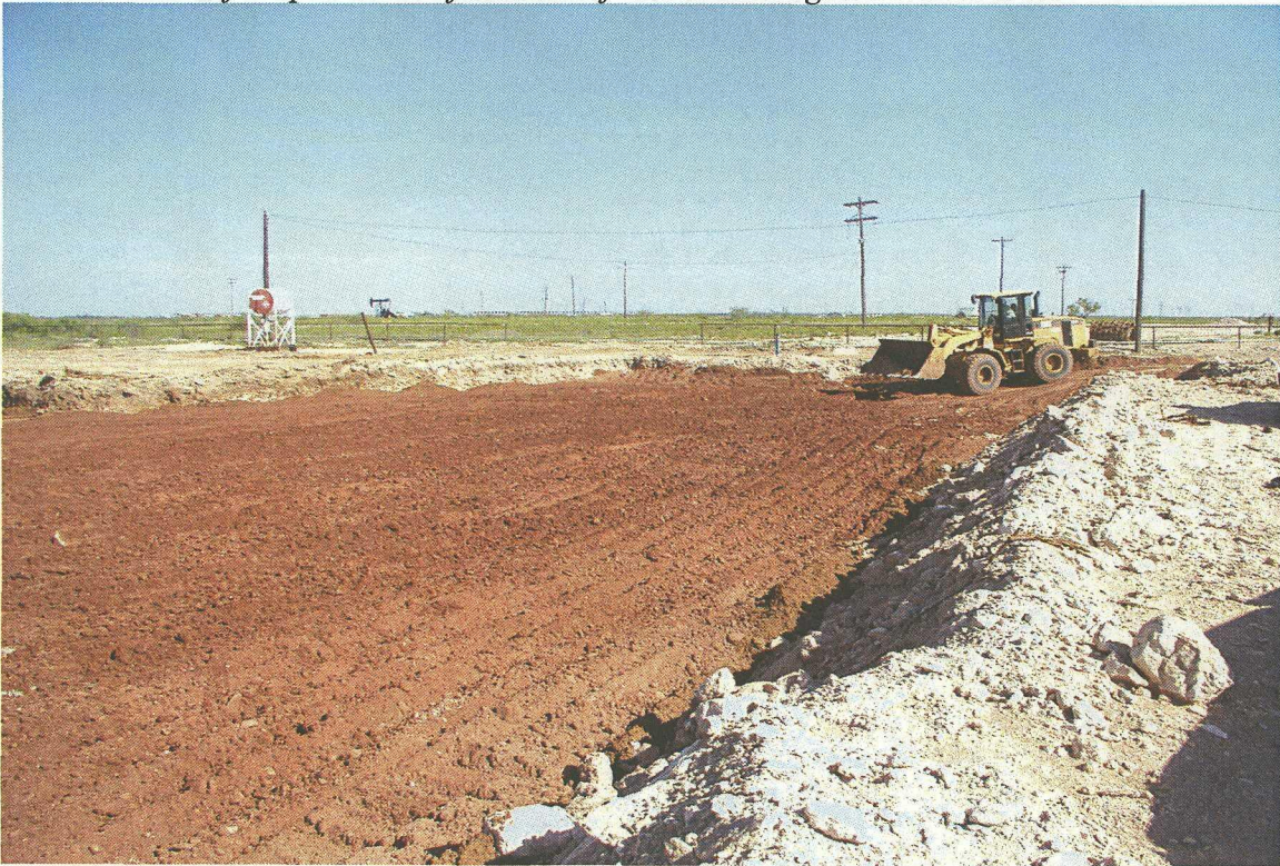
No. 102 – View of compaction in the northeast excavation area while processing the sand material.
