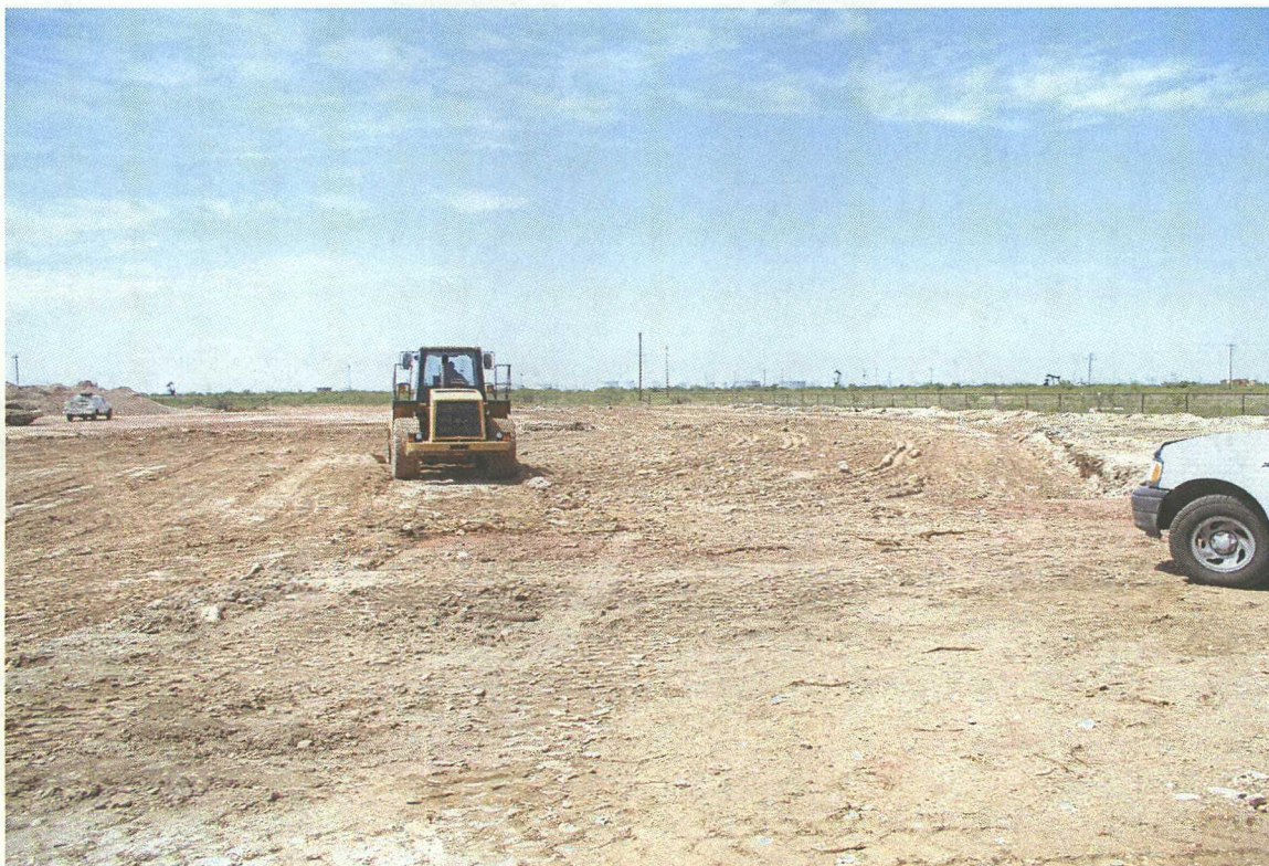
No. 107 – View of caliche material being installed in the large excavation area.
