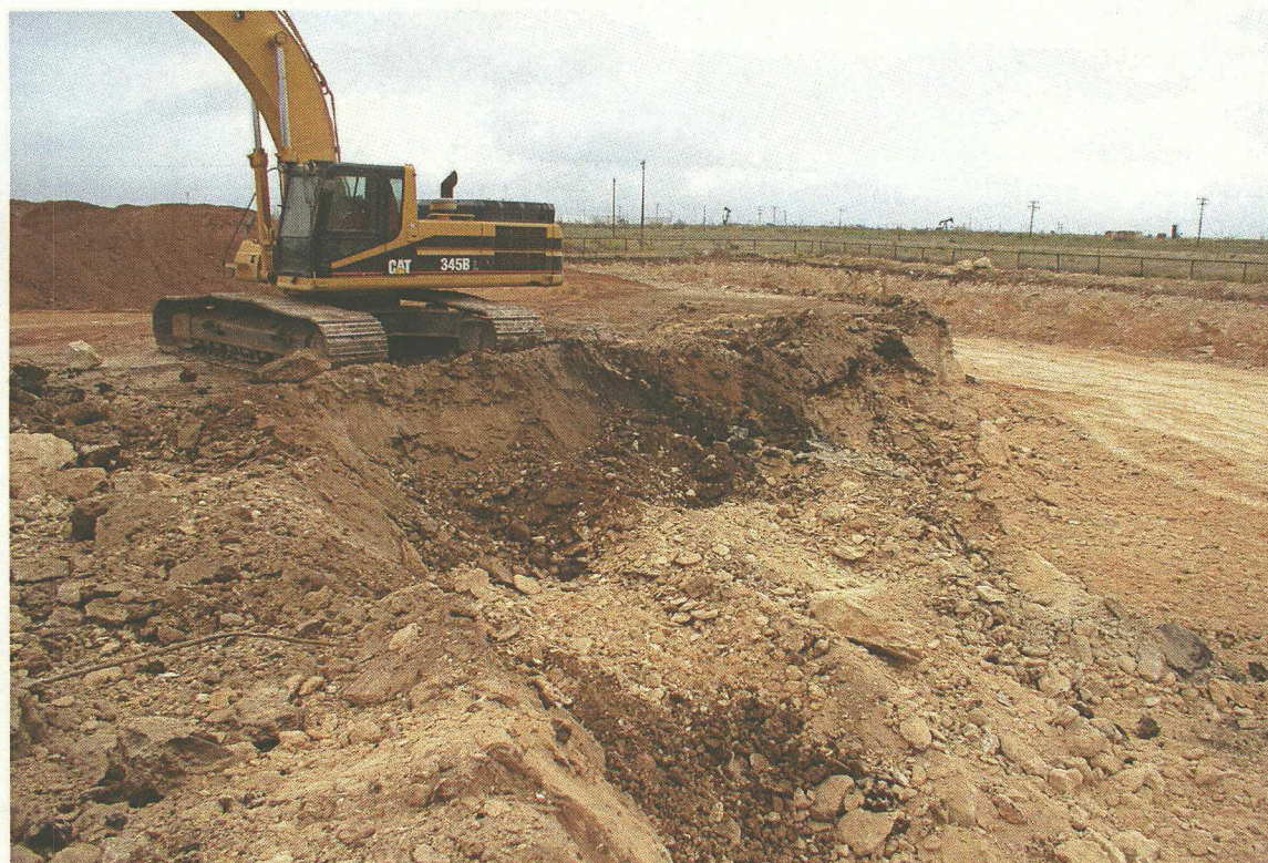
No. 40 – View of continuing excavation to 10 feet below ground surface.
