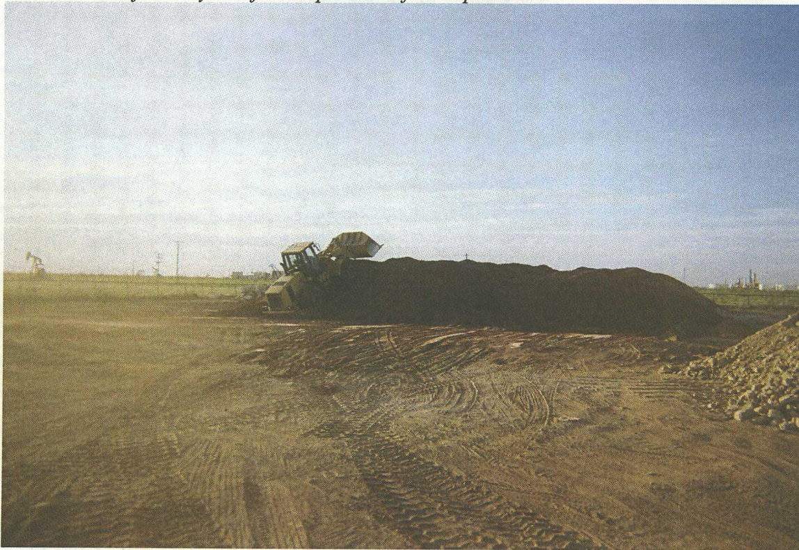
No. 18 – View of the clay backfill being pushed up to maximize room on site.
