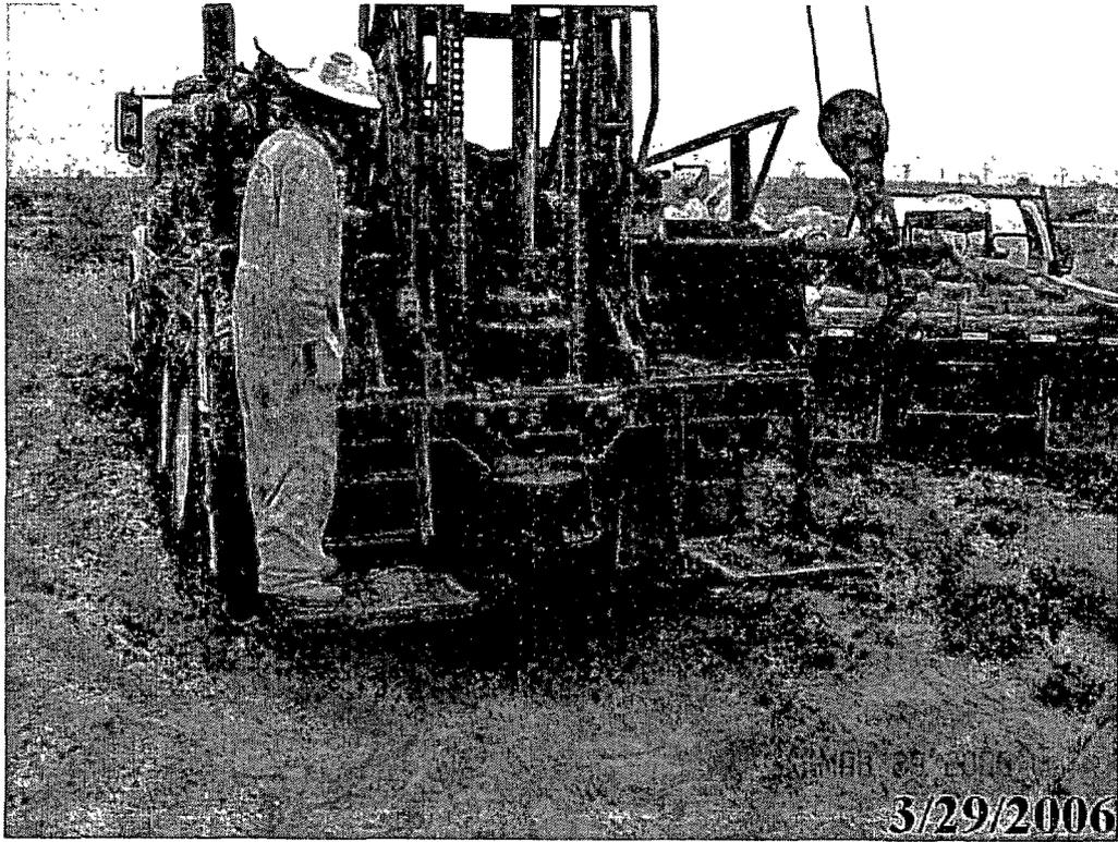
**Photo #9:** Installation of Monitor Wells.
