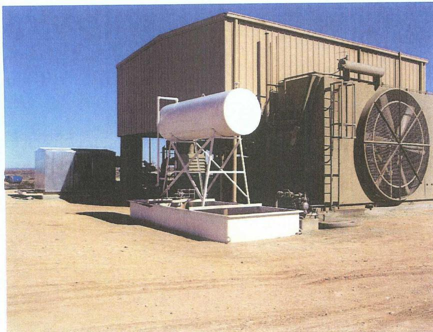
*Figure 7: 1000 Gallon Steel Lubrication Oil Tank TK-5 and 1100 Gallon Steel Secondary Containment (note vault for TK-6 by lower right corner of TK-5 containment).*
