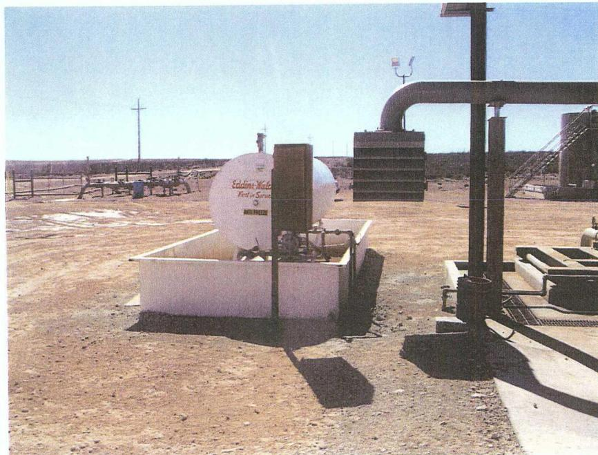
*Figure 6: 1000 Gallon Steel Antifreeze Tank TK-4 and 1100 Gallon Steel Secondary Containment.*
