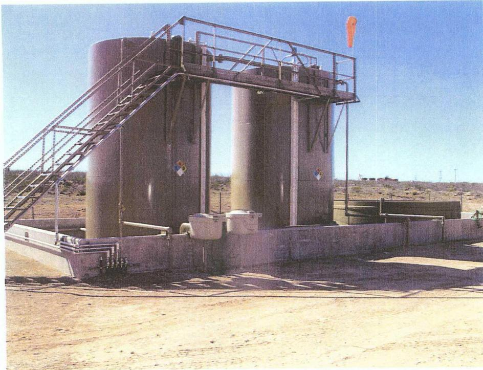
*Figure 5: 210 Barrel Tanks TK-1, TK-2 and 100 Barrel Tank TK-3 (left to right) and concrete secondary containment structure.*
