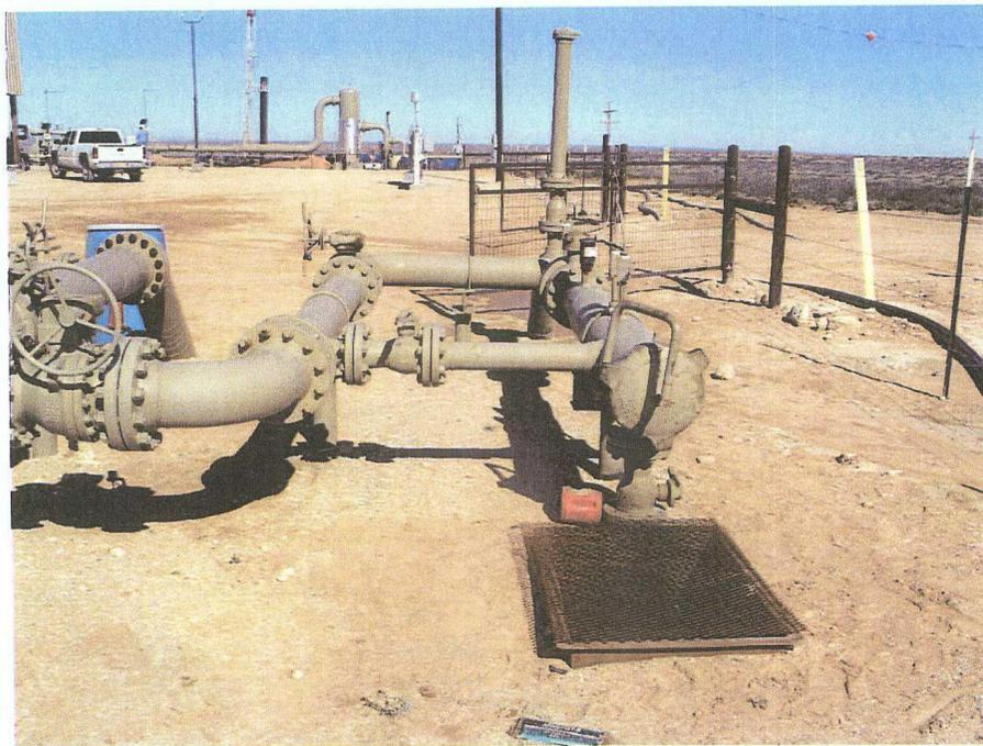
*Figure 11: Pig Waste Steel Containment TK-8*
