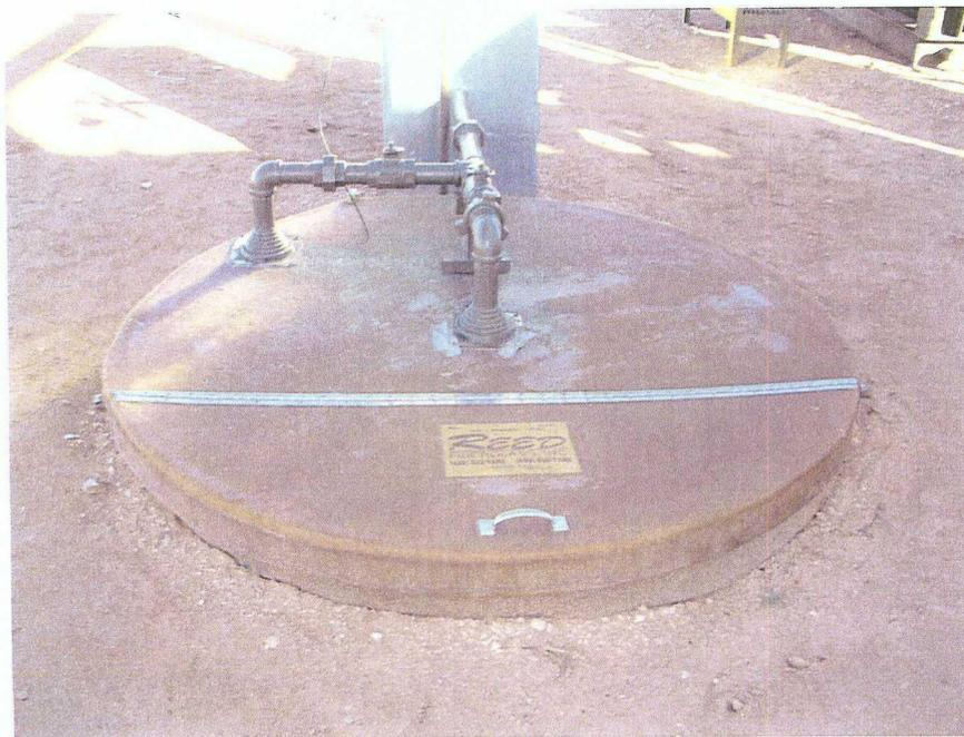
*Figure 8: Top Cover of Double Walled Fiberglass Vault Holding Waste Oil Tank TK-6*
