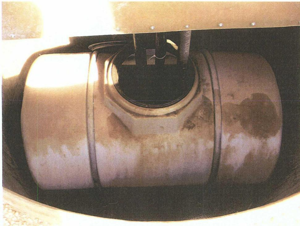
*Figure 10: Waste Oil Tank TK-8 in Subgrade Fiberglass Containment*
