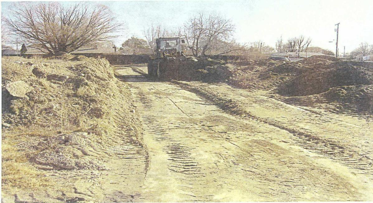
Viewing east near central portion of the former Aerex site. Soil stockpiles were moved to allow access for direct push grid locations. Stockpiled soils apparently were placed onsite from excavation for road construction along adjacent Blanco Boulevard.
