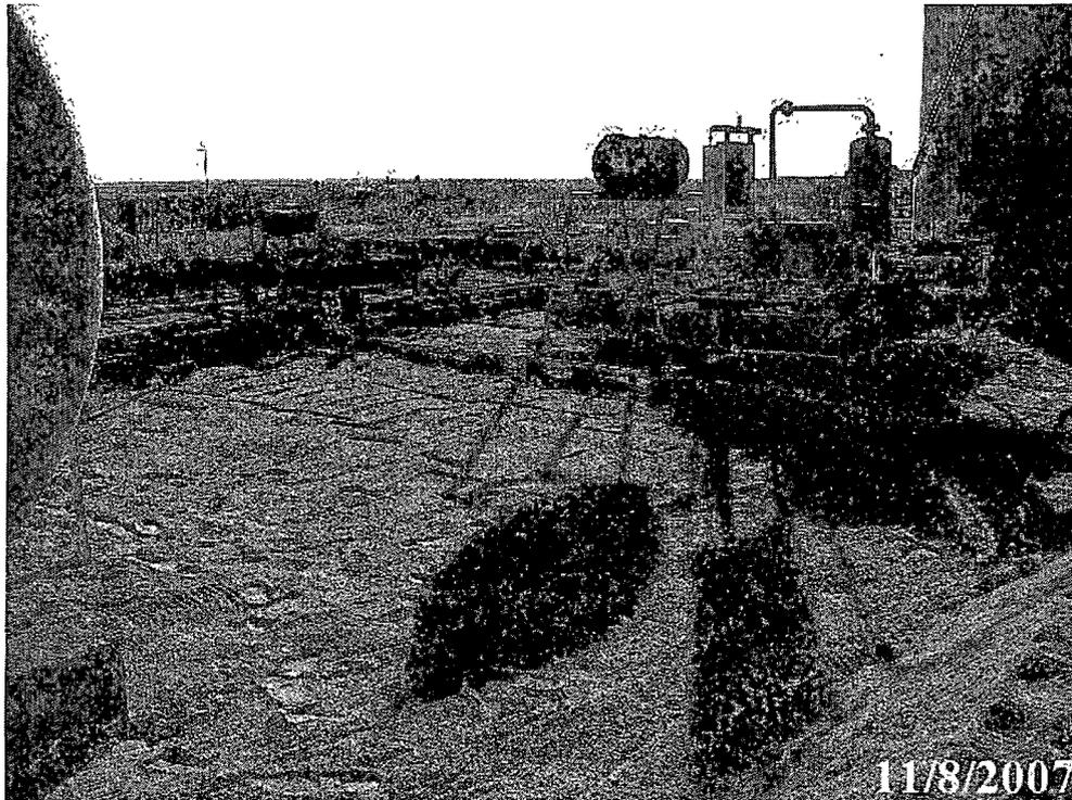
Photograph No. 8 – Remediated site showing graded caliche backfill material
