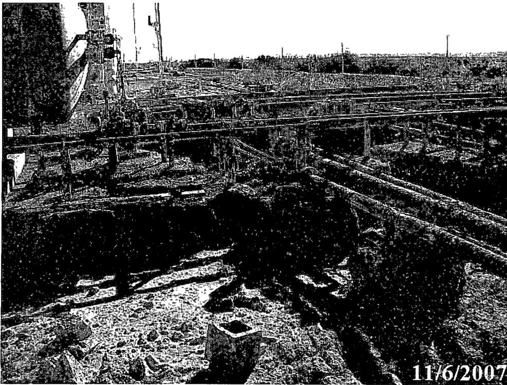
Photograph No. 6 – Excavation area showing piping, horizontal separator and earthen supports
