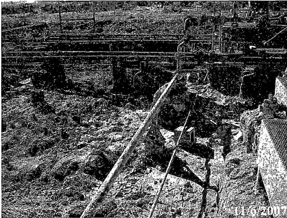
Photograph No. 5 – Excavation area and piping with earthen supports.
