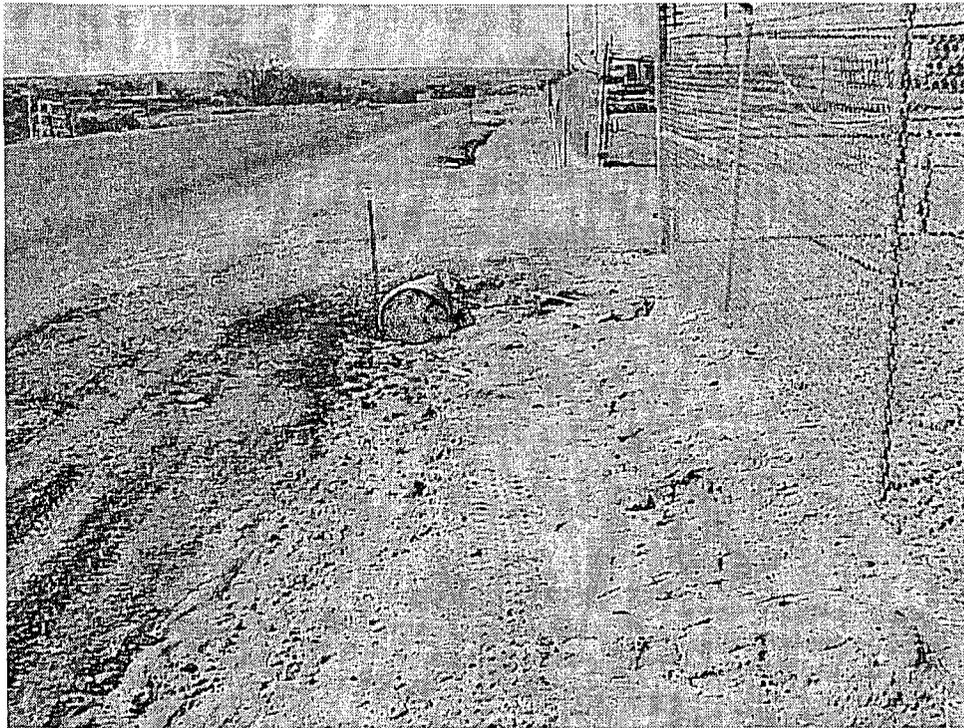
WO # 57873 Please repair the culvert located @ southeast entrance from Sullivan Rd. to burner rack. It has been run over
