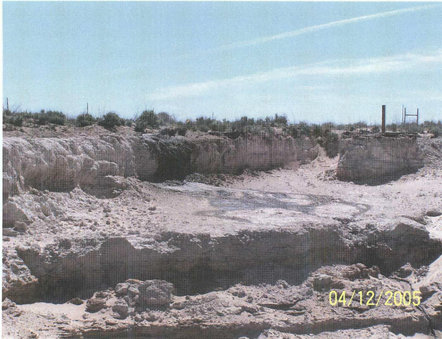
Photograph #9- Looking westerly at Sid Richardson release. Dark stained soil is natural gas liquid contaminated soil.
