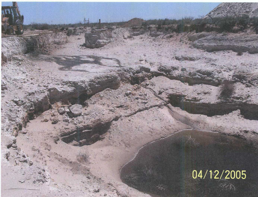
Photograph #10- Looking southerly at Sid Richardson release. Dark stained soil is natural gas liquid contaminated soil.
