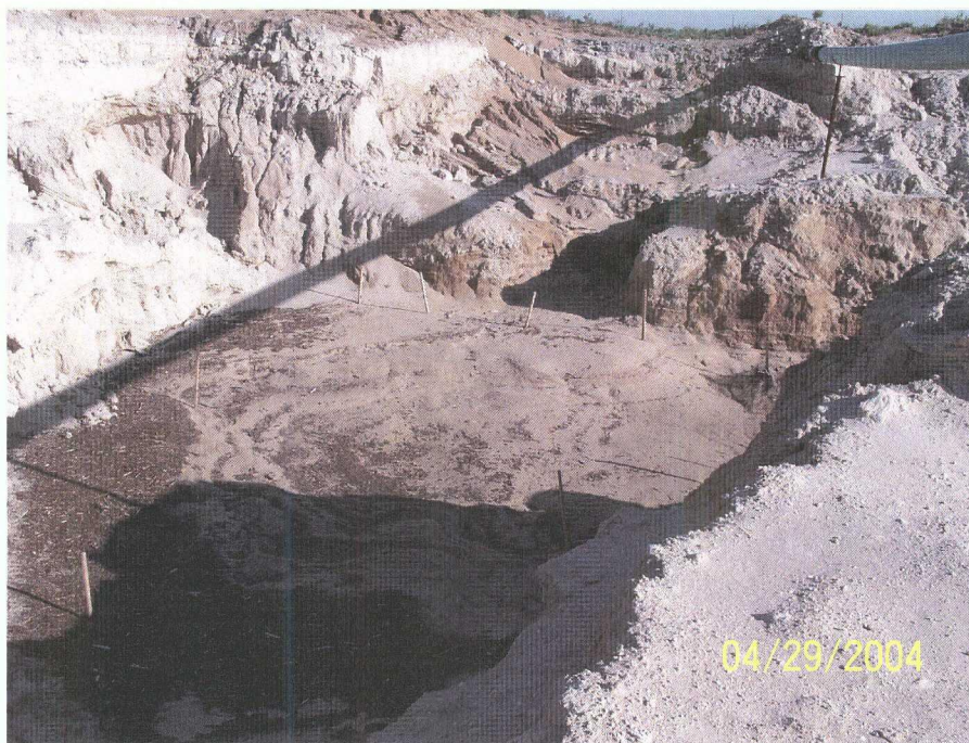
Photograph #7- Looking southerly at excavation.
