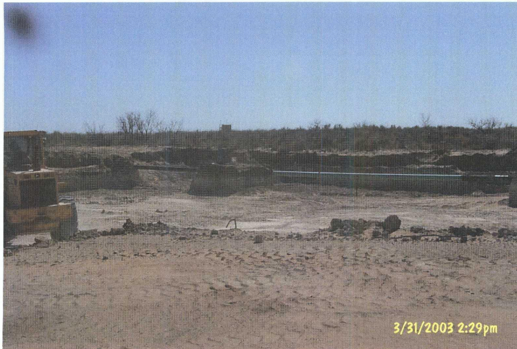
Photograph #3- Looking westerly at excavation activities.
