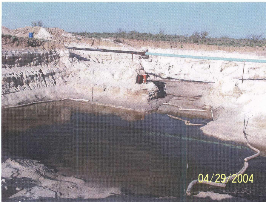
Photograph #6- Looking westerly at excavation.
