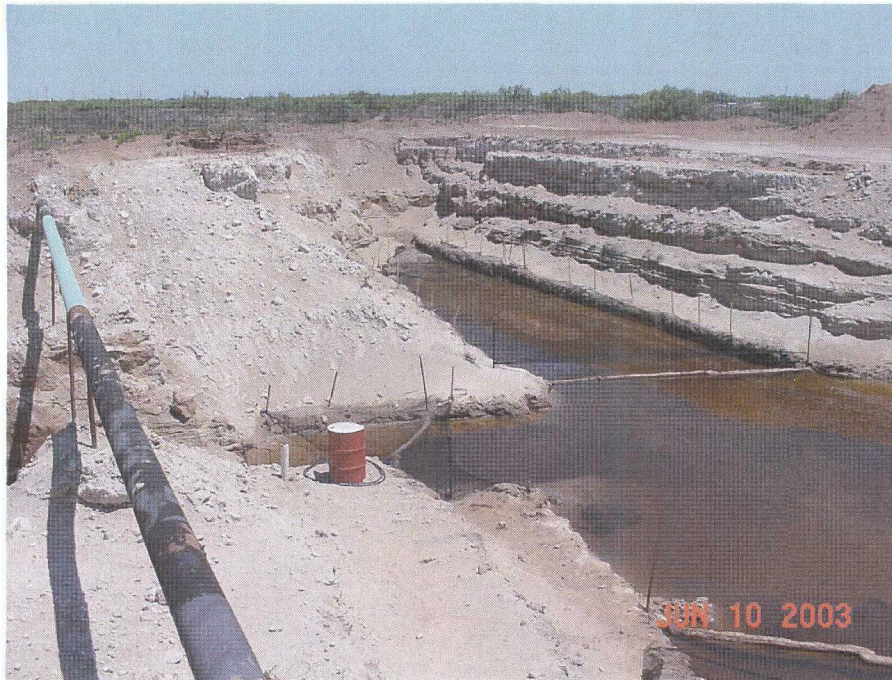
Photograph #5- Looking northerly at excavation.
