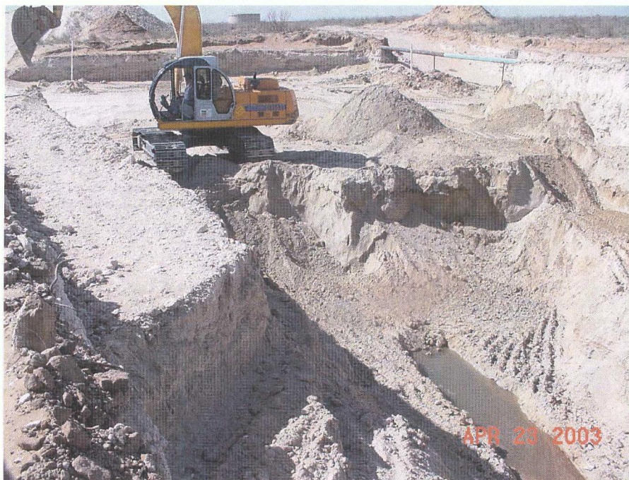
Photograph #4- Looking southerly at excavation activities.
