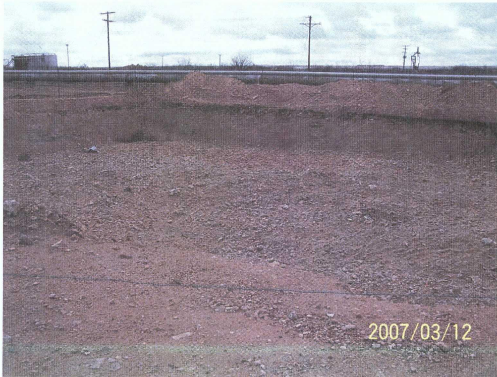
Photograph #3 – Looking at northeast corner of pit excavation
