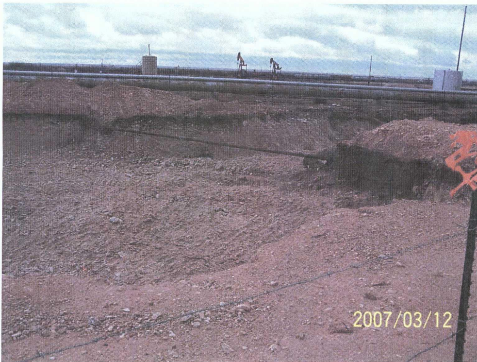
Photograph No. 4 – Looking at southeast corner of pit/northwest corner of overflow area
