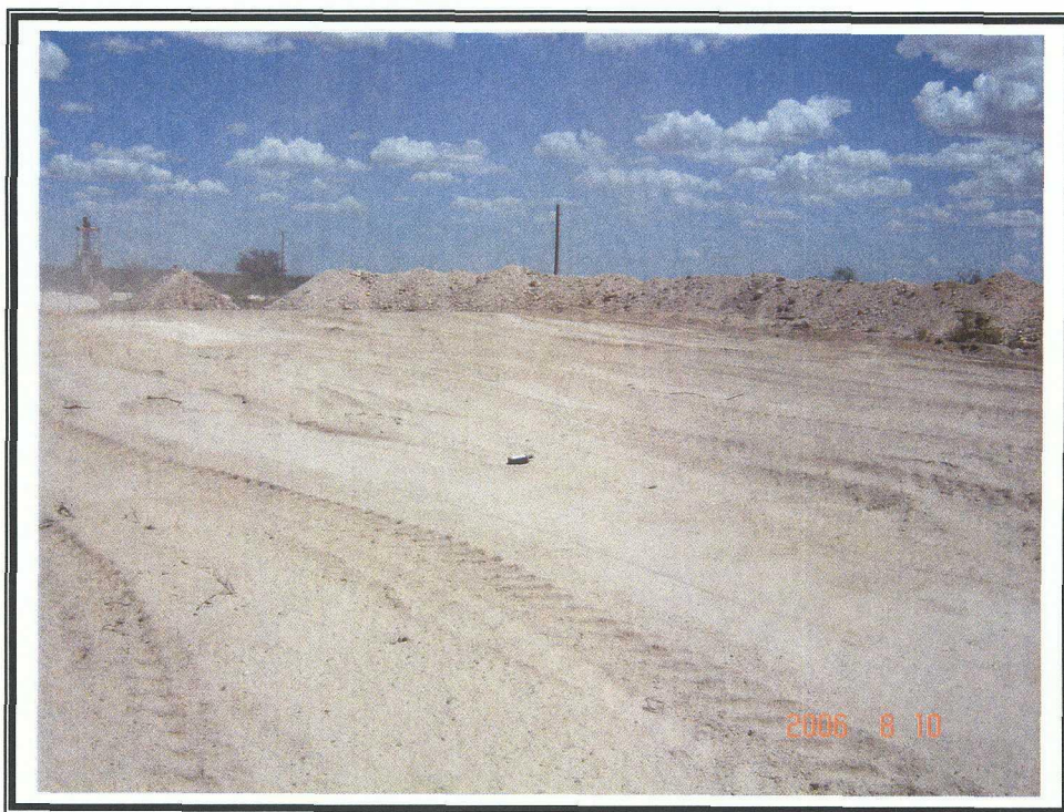
Texaco State "G" Lact Unit Battery #22 backfill of Burn Pit complete
