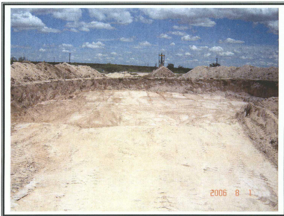
Texaco State "G" Lact Unit Battery #22 Burn Pit backfill of fines to 6' bgs
