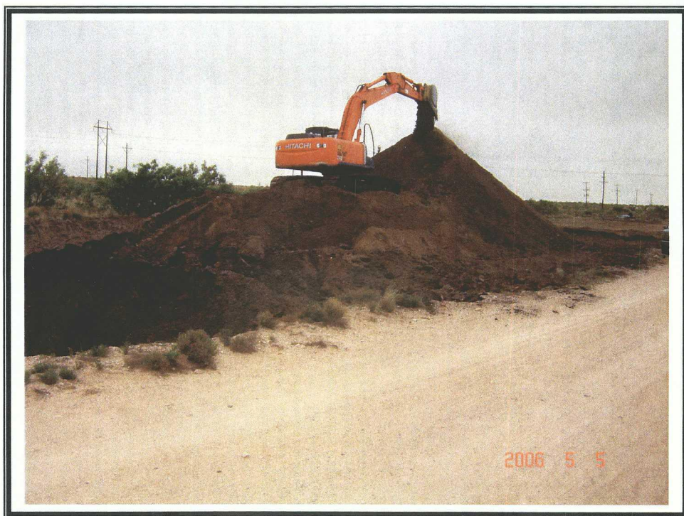
Texaco State "G" Lact Unit Battery #22 excavation of Burn Pit
