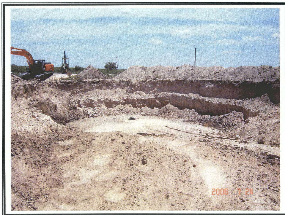
Texaco State "G" Lact Unit Battery #22 excavation of Burn Pit rim
