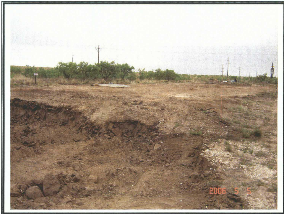
Texaco State "G" Lact Unit Battery #22 Tank Battery Area
