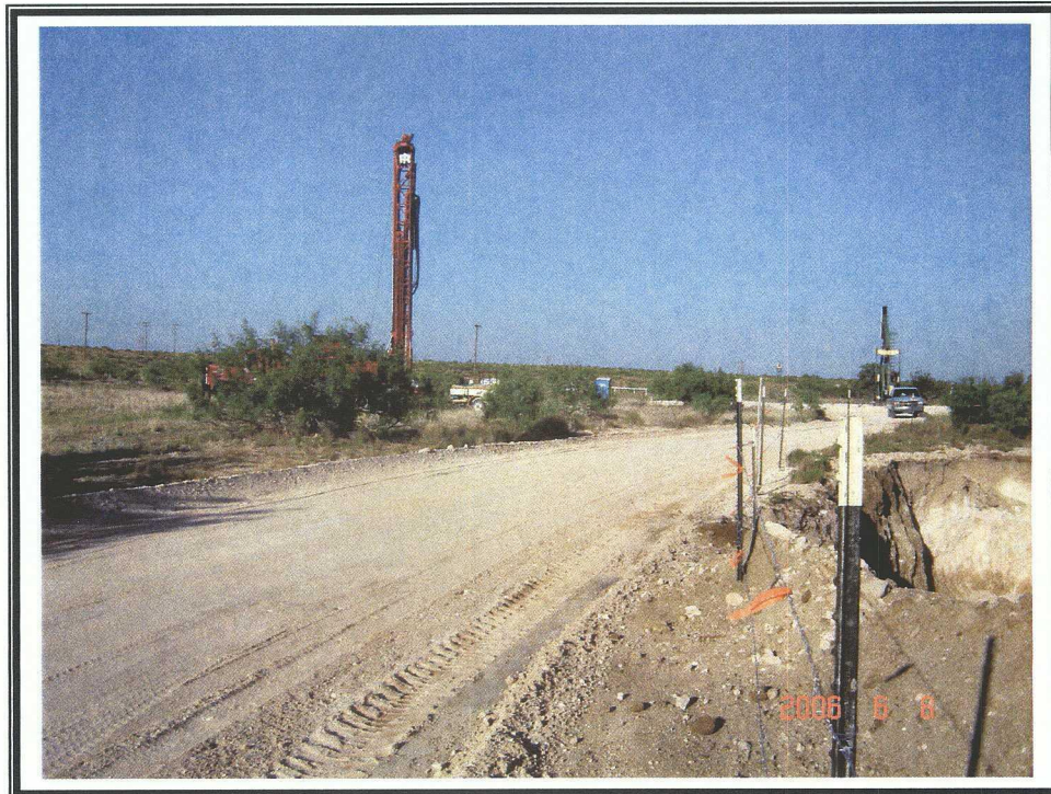
Texaco State "G" Lact Unit Battery #22 drilling of MW2
