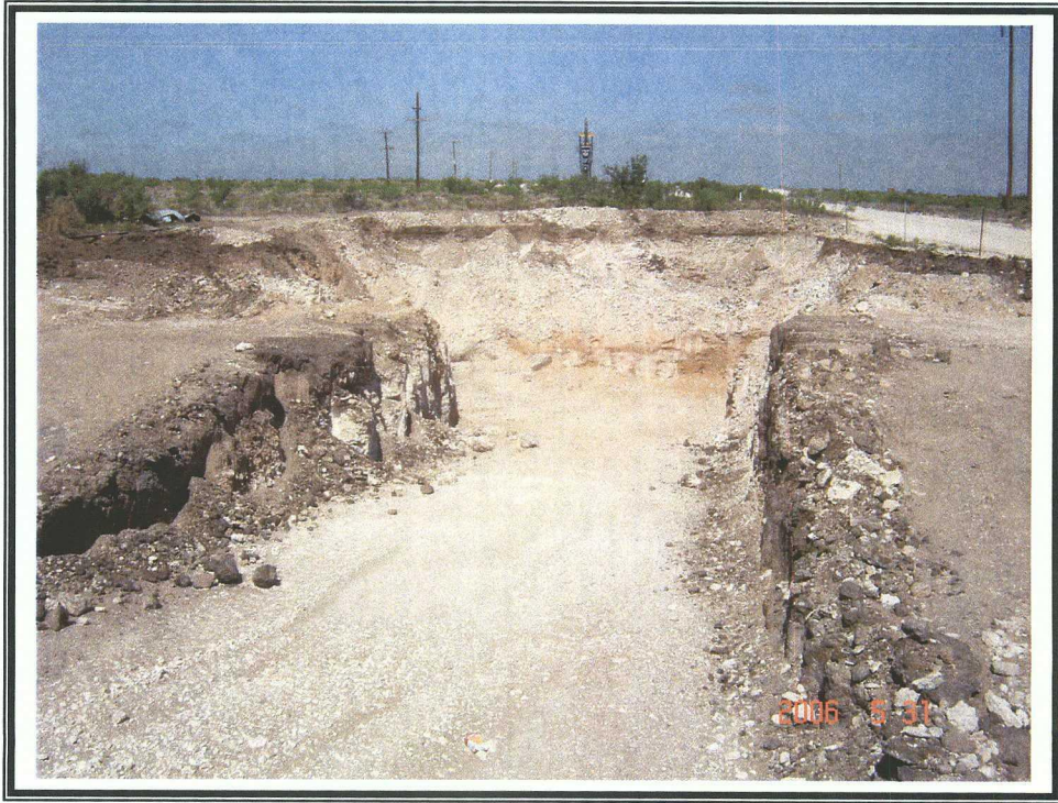
Texaco State "G" Lact Unit Battery #22 Battery Excavation
