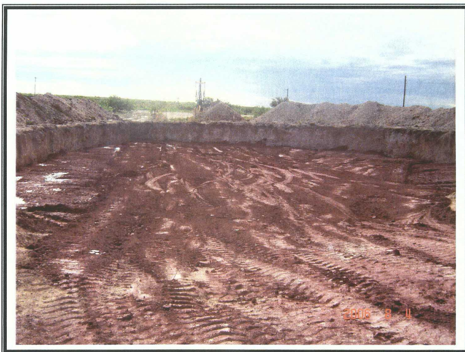
Texaco State "G" Lact Unit Battery #22 Burn Pit installation of clay liner
