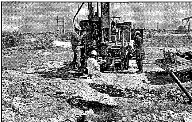
*Figure 1: Soil boring taken May 2, 2006 immediately over the former junction box at the B-32 site.*
