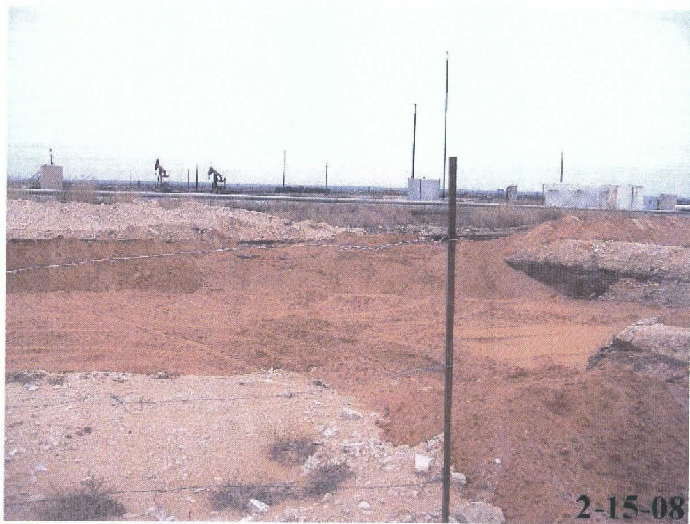
Photograph No. 8 – Backfilling excavation.
