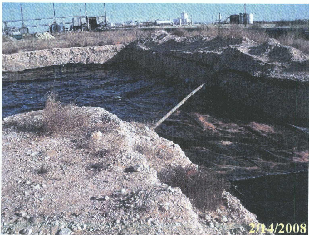
Photograph No. 7 – Installation of liners.
