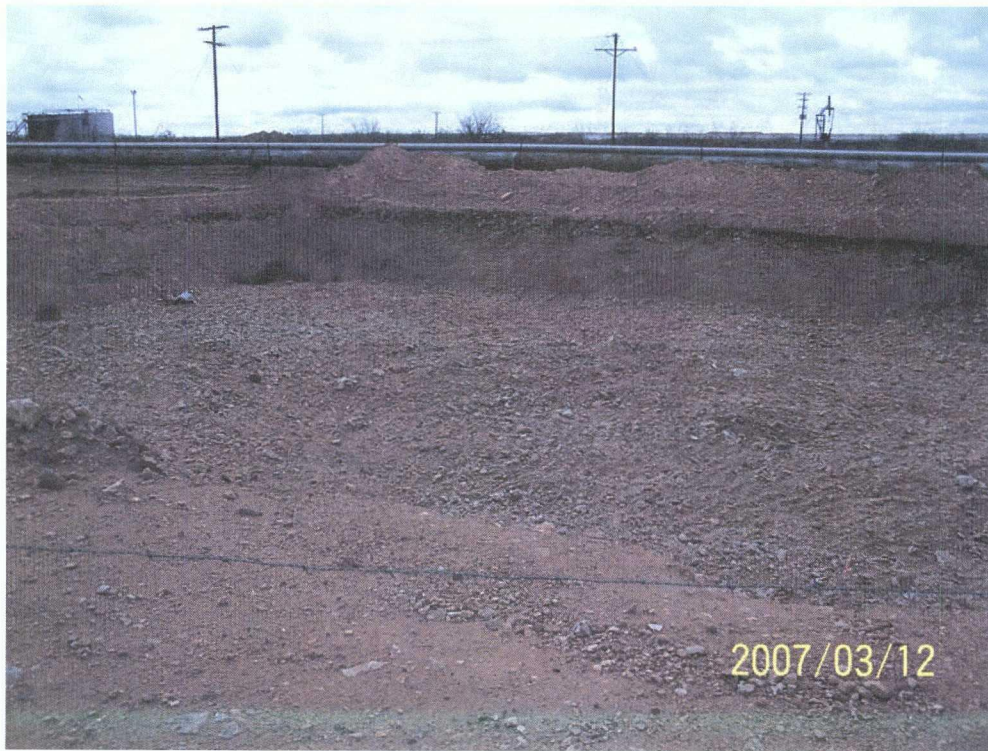
Photograph No. 3 – Looking at northeast corner of pit excavation.
