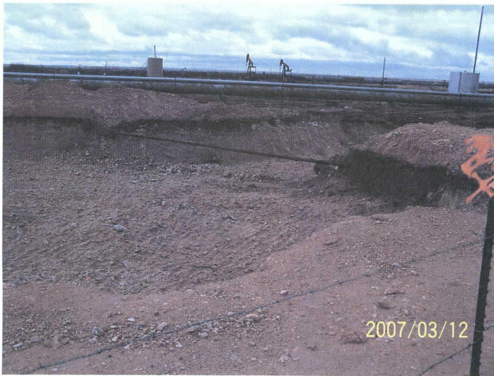
Photograph No. 4 – Looking at southeast corner of pit/northwest corner of overflow area.
