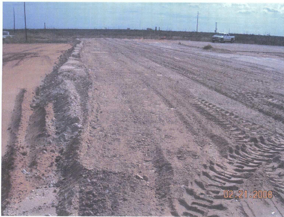
Photograph No. 10 – Remediated site.
