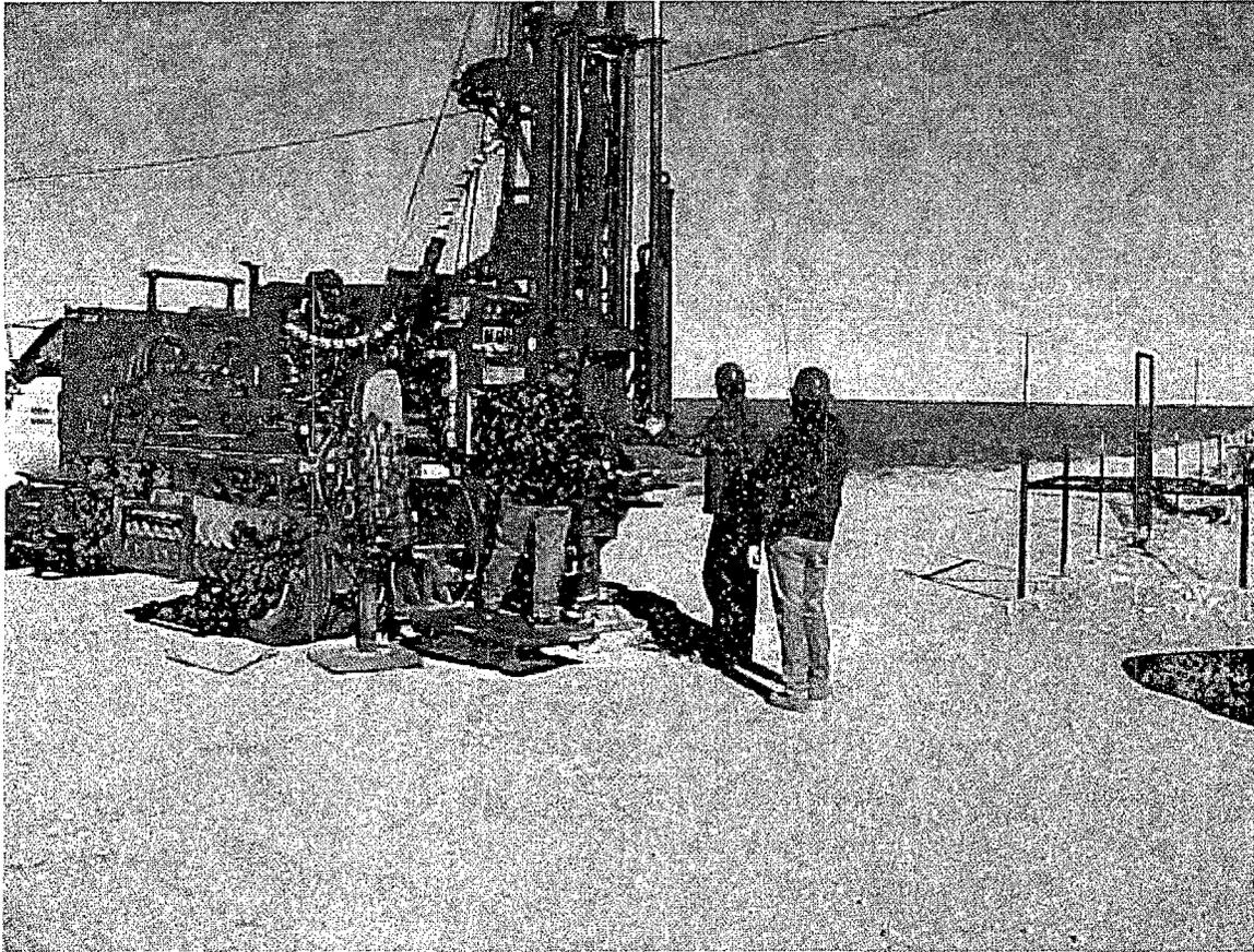
Drilling of SB-3A, southwest corner outside bermed area on 11/20/03. Soil borings 3 and 3A are drilled in the same location within 2' feet of each other.
