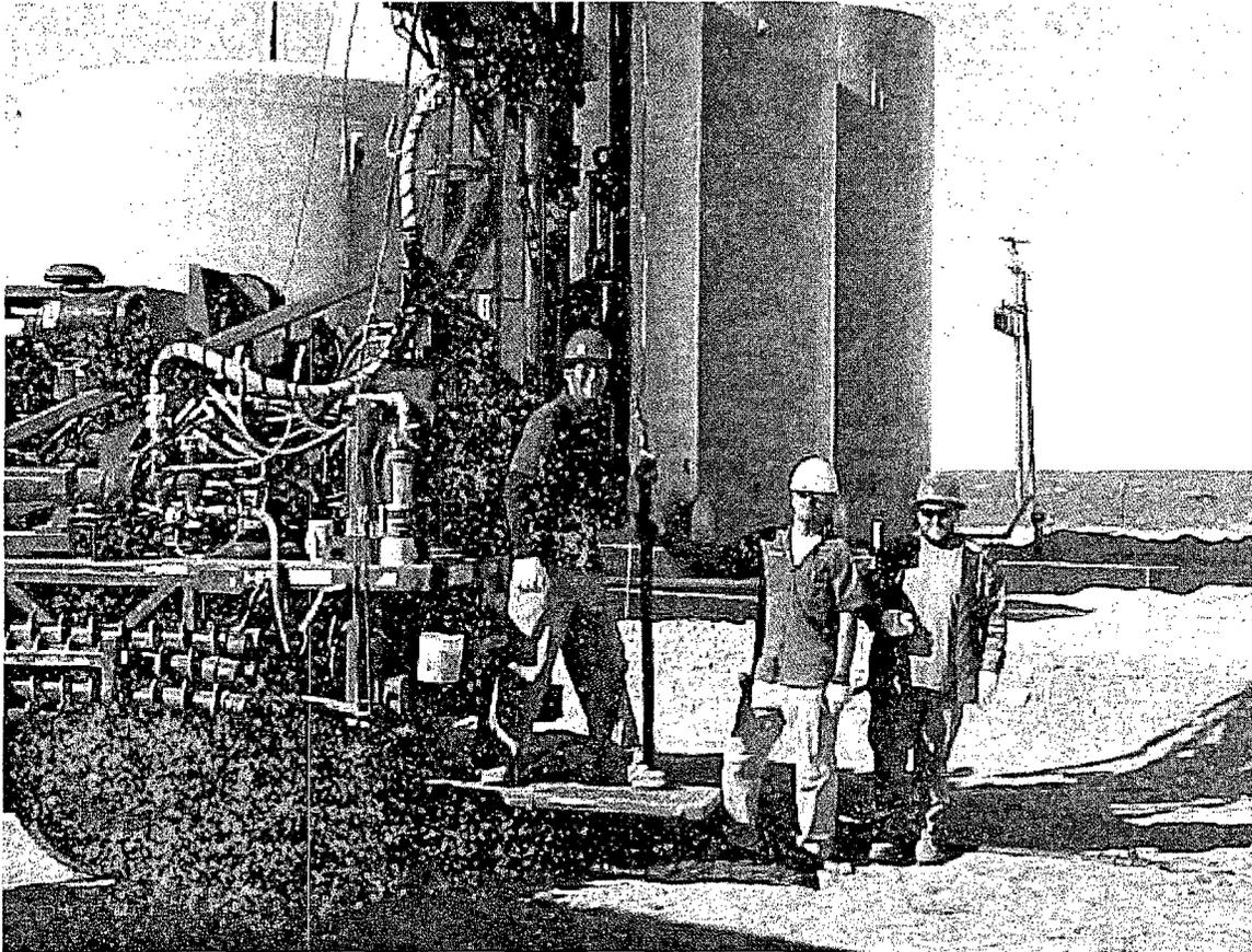
Location of Soil Boring SB-1 NMSWDCO, October 14, 2003, east side of the new tank battery and reworked berm area surrounding the tank battery. Drilling Rig is Mobile Drill B-58 Owned by Atkins Engineering Associates, Roswell, New Mexico. Total Depth 11' feet below ground surface.
