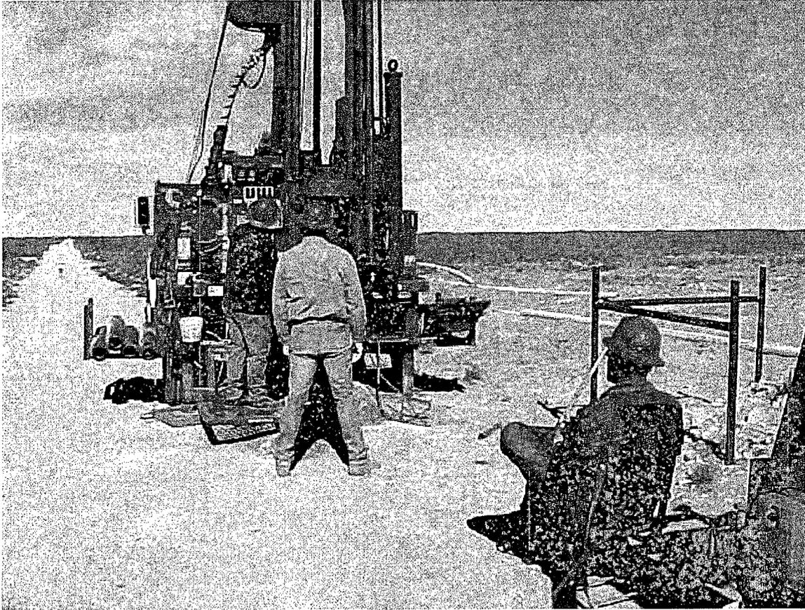
Drilling of SB-4A, northwest corner outside bermed area on 11/20/03. Soil borings 4 and 4A are drilled in the same location within 6' feet of each other.
