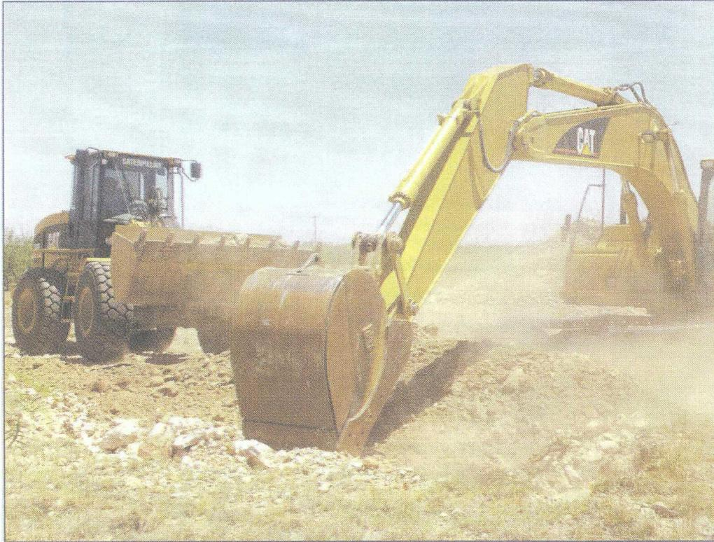
*No. 1 – Beginning to excavate the overburden from the 2007 excavation.*
