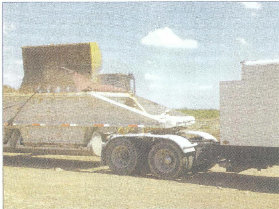
*No. 4 – Loading a belly dump truck to haul the contaminated soil to the CRI facility.*
