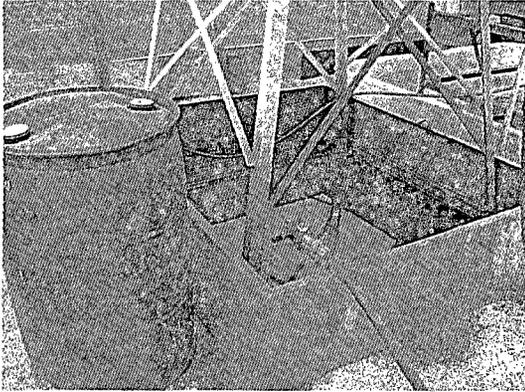
Photo 1: Secondary containment holding fluids with soil staining near outer rim of containment.
