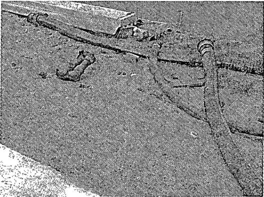
Photo 9: Engine wash area flush directly on ground.
