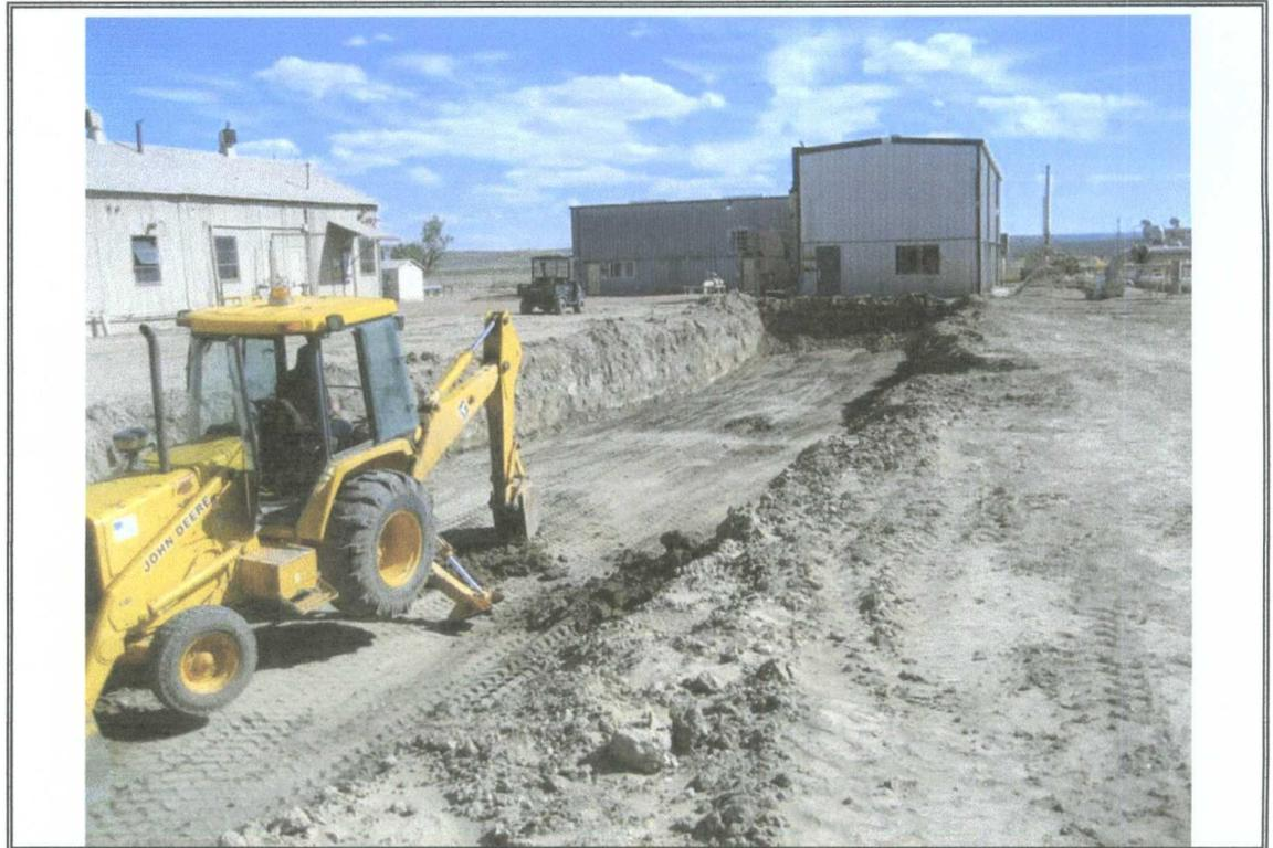
Photograph Number 9: View of backhoe performing vertical extent in the center of the trench 120' north of the Saturn Building
