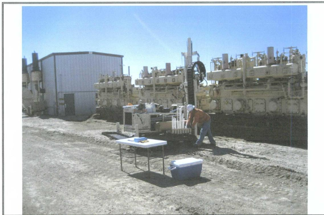
Photograph Number 7: View of the geprobe performing soil borings on the east side of the Clark Compressors.
