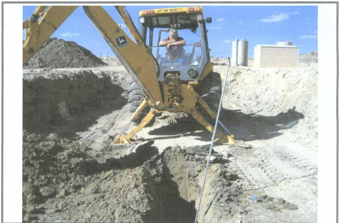
Photograph Number 10: View of backhoe performing vertical extent in the center of the trench 120' north of the Saturn Building
