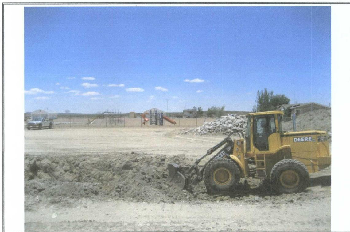
Photograph Number 4: View of the excavation of the Clark foundation trench.
