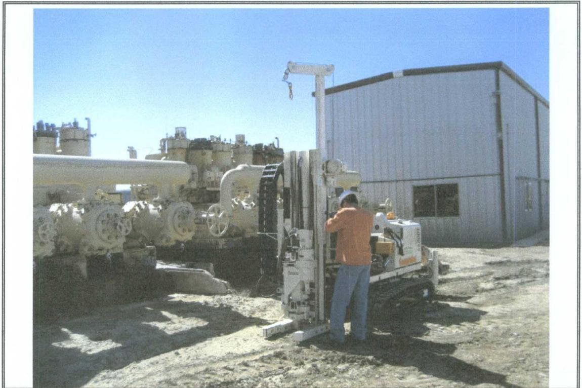
Photograph Number 1: View of the geoprobe direct push unit performing borings at the southwest corner of the former Clark compressor building in the (vicinity of SB2W).
