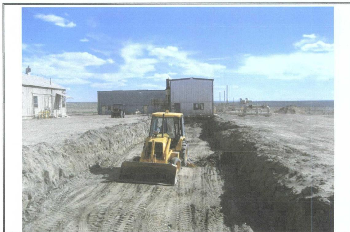
Photograph Number 8: View of backhoe performing vertical extent in the center of the foundation trench.
