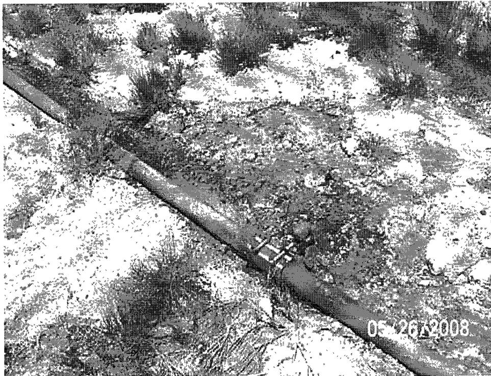
Photograph No. 2 – Point of release and clamp
