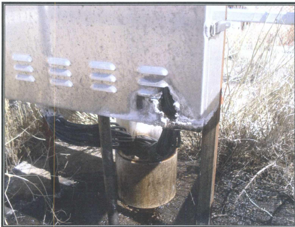
Photo2: Damage to Cathodic Well system
