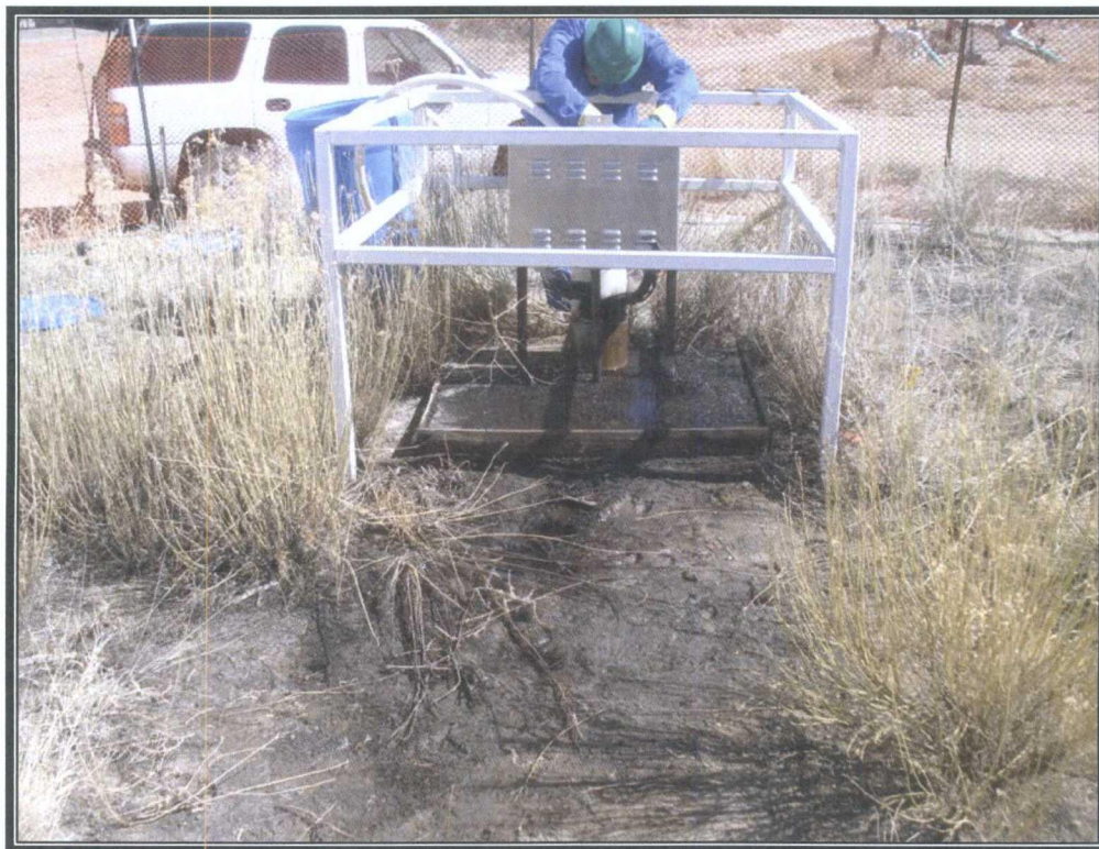
Photo 1: Installation of acid collection system
