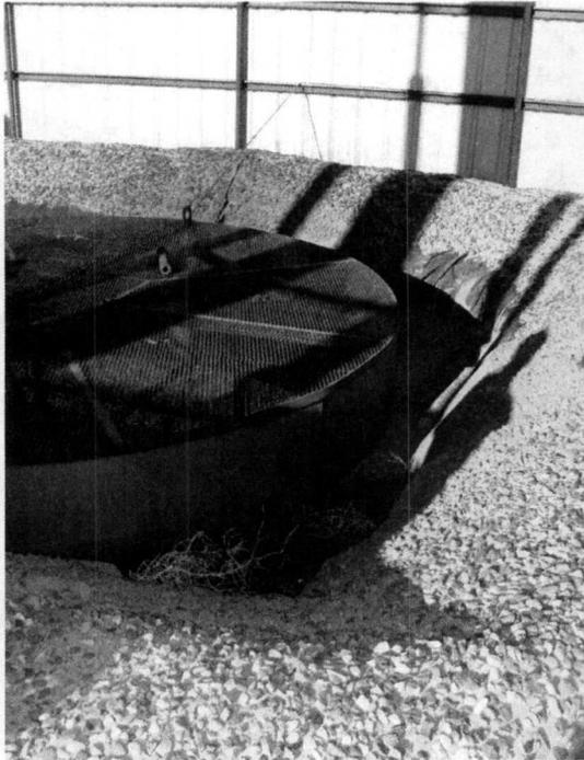
Photo 2: BGT-1 with sediment in secondary containment area.
