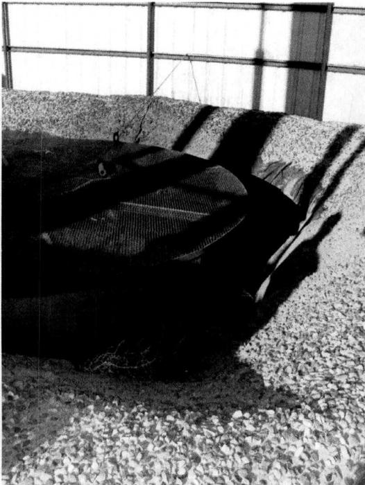
Photo 2: BGT-1 with sediment in secondary containment area.
