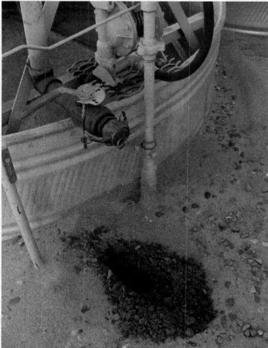
Photo 7: Saddle tank area with discharge conduit outside of secondary containment. Soil staining.
