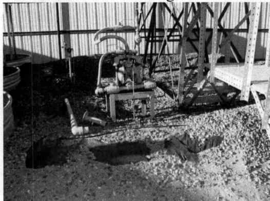
Photo 8: Eroded bermed area.
