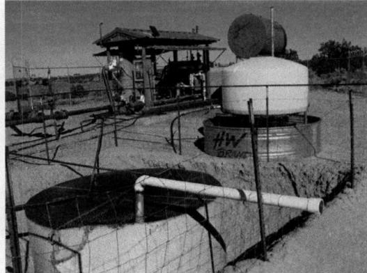
Photo 5: Single wall BGT with compressor in background.
