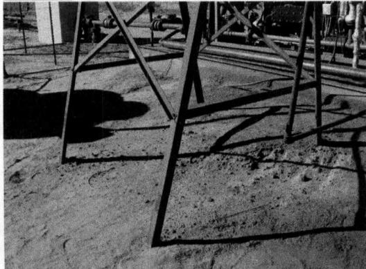
Photo 2: No secondary for saddle tank.
