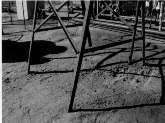
Photo 2: No secondary for saddle tank.
