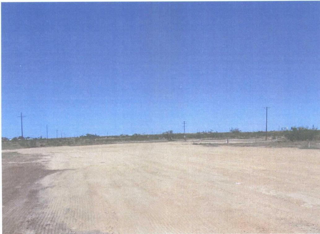
Looking North, Remediation Completed, Excavation Backfilled, Contoured and Seeded
