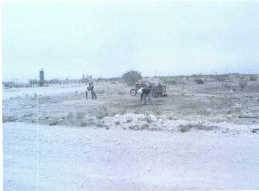
4/28/09: REMOVING LARGER ROCKS FROM AREA
