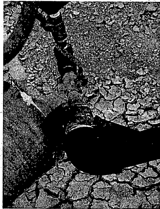
Recommended AFE to replace 1/2 inch dia. pipe with 1 inch or greater.
