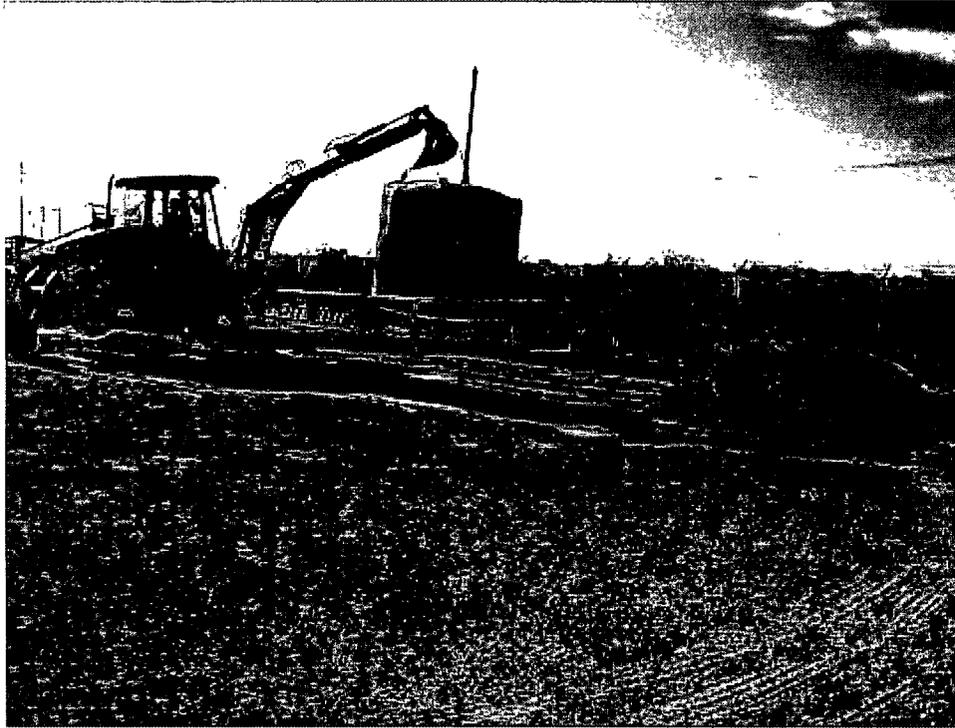
View Facing SSW: Backhoe Removing Tank 2 from Excavation
