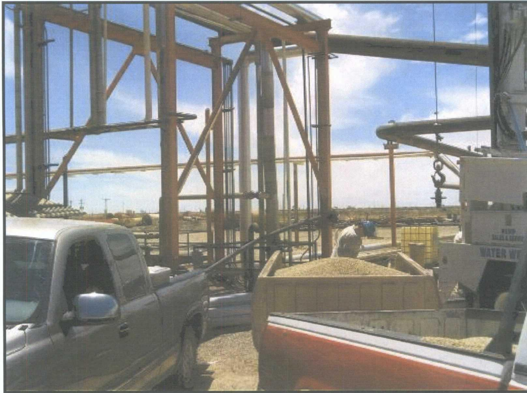
Gravel fines for well. Screen length 30 feet, gravel above screen for oil recovery, April 2009
