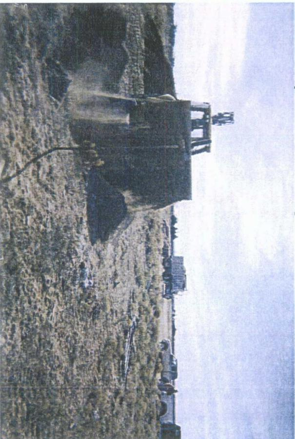
backfilling excavation with clean, imported soil in background, facing southwest
