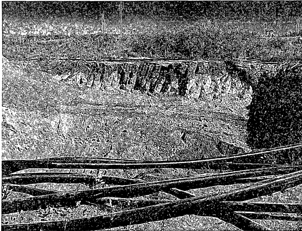
Facing east across pasture after excavation 8-15-09
