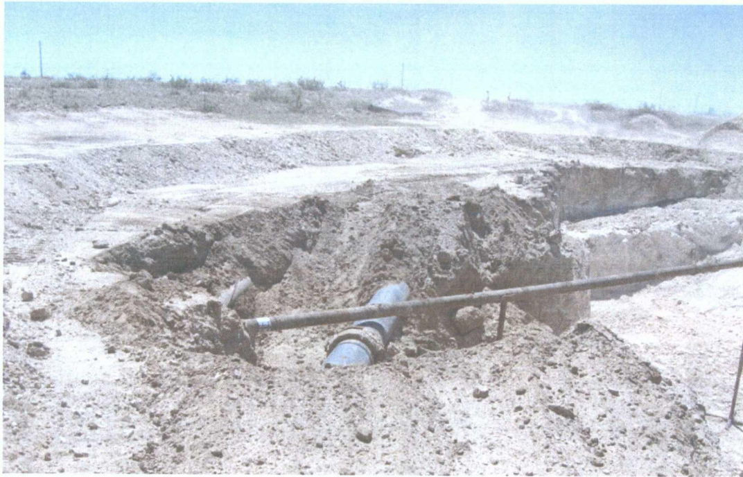
DCP Plant to Lea Station 6-Inch Sec 31 excavation, looking southeast
