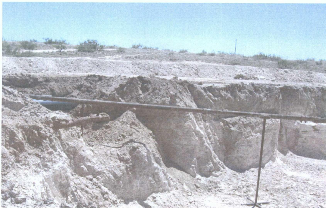
DCP Plant to Lea Station 6-Inch Sec 31 excavation, looking east
