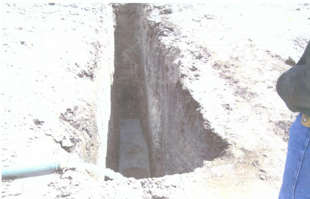
DCP Plant to Lea Station 6-Inch Sec 31, North Trench #1 and East Trench #1 Soil Amendments being placed in Trenches
