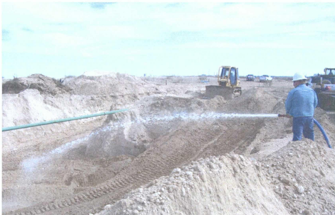
DCP Plant to Lea Station 6-Inch Sec 31 excavation, water packing backfill material
