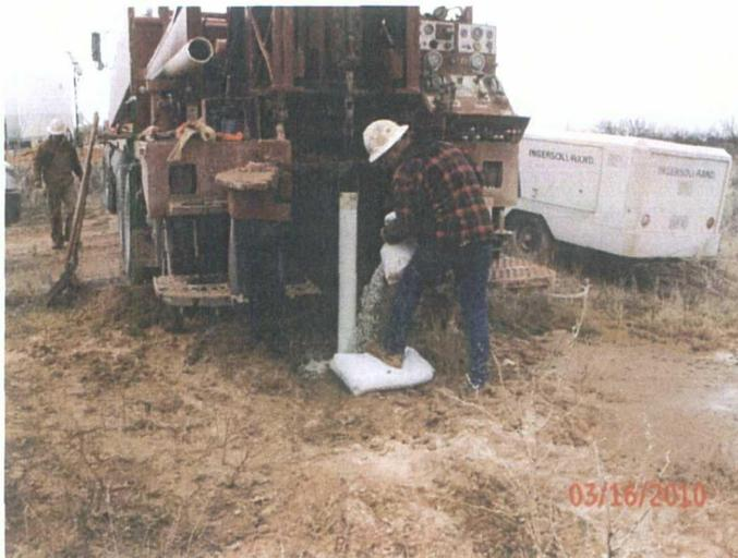
Sealing the well with bentonite
