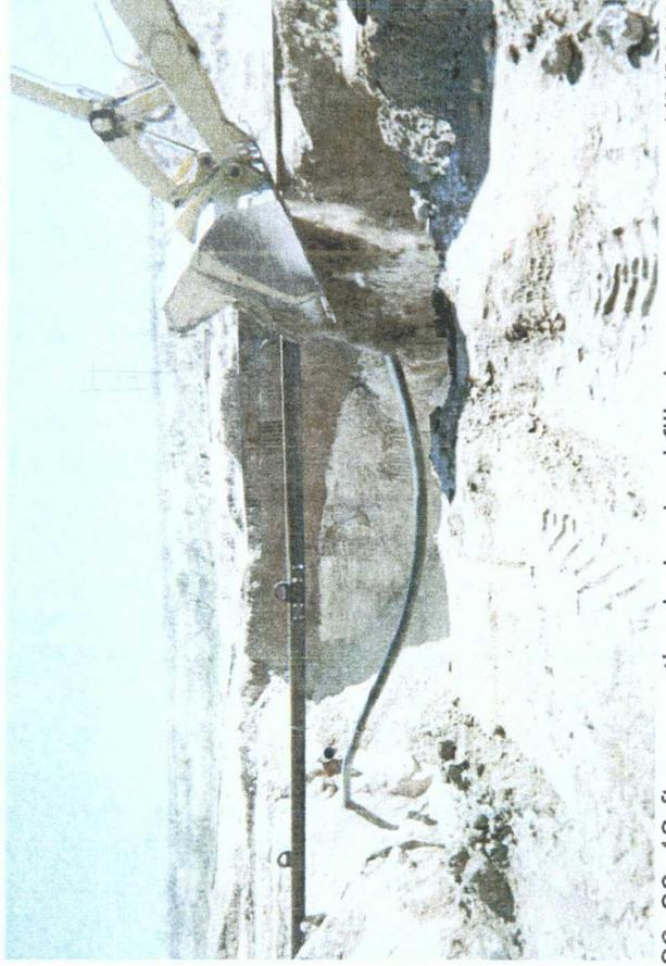
20x20x12-ft excavation being backfilled
