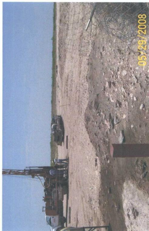
View facing west showing drilling/sampling at soil boring B-3 located about 25 south of drilling pit. Monitoring well MW-1 is shown in foreground.
