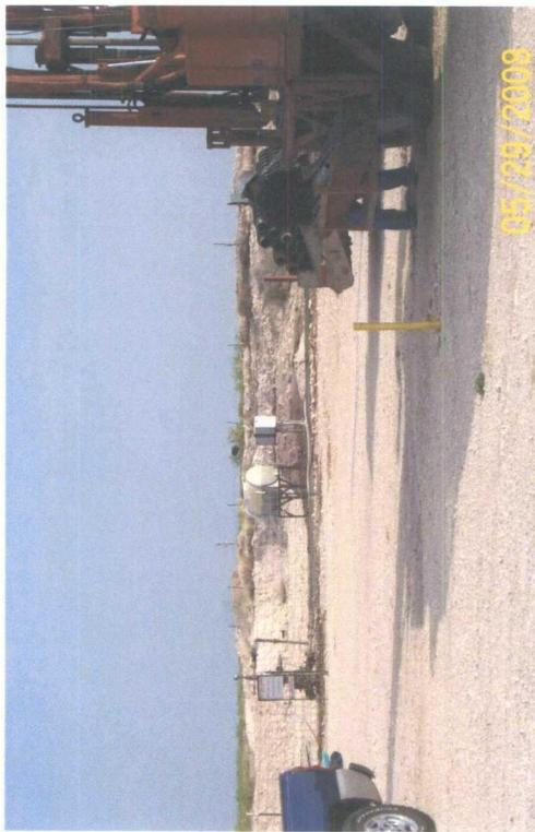
View facing northwest showing drilling activities at soil boring B-1. Wellhead and drilling pit shown at left-center.
