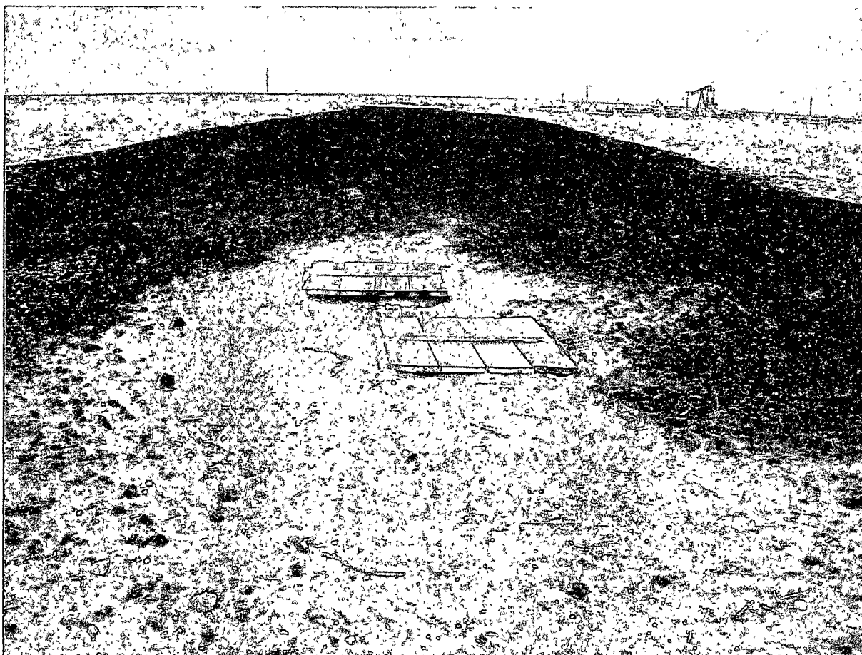
Melrose St. 647-711 #89 p/l leak Photo viewing: from the nne. to sw. Close up view of junction boxes for valves
