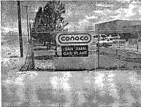
Pic #1-Plant Entrance
